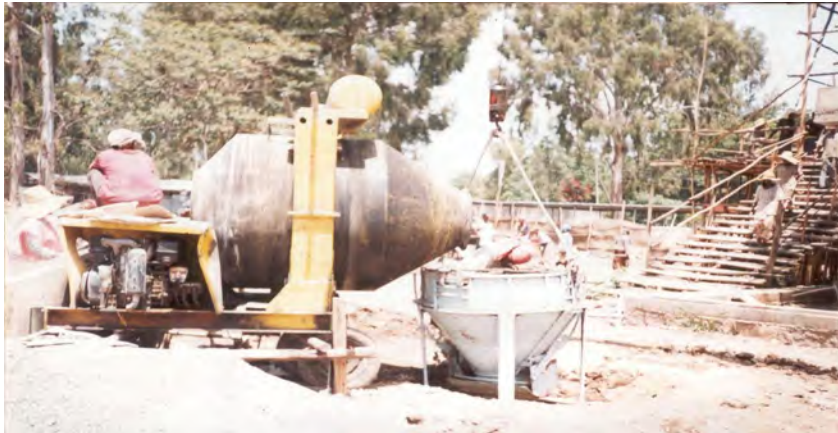
b. Picture of 750 liters concrete mixer discharging the mixed concrete
