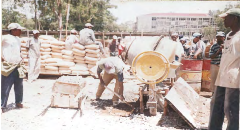
a. Picture of 250 liters stationary concrete mixer being batched
