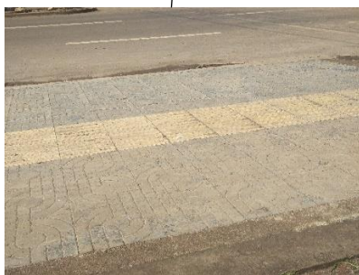
Fig 4.2c Typical 30m asphalt road with side walkway paved with tile and greenery at the median
