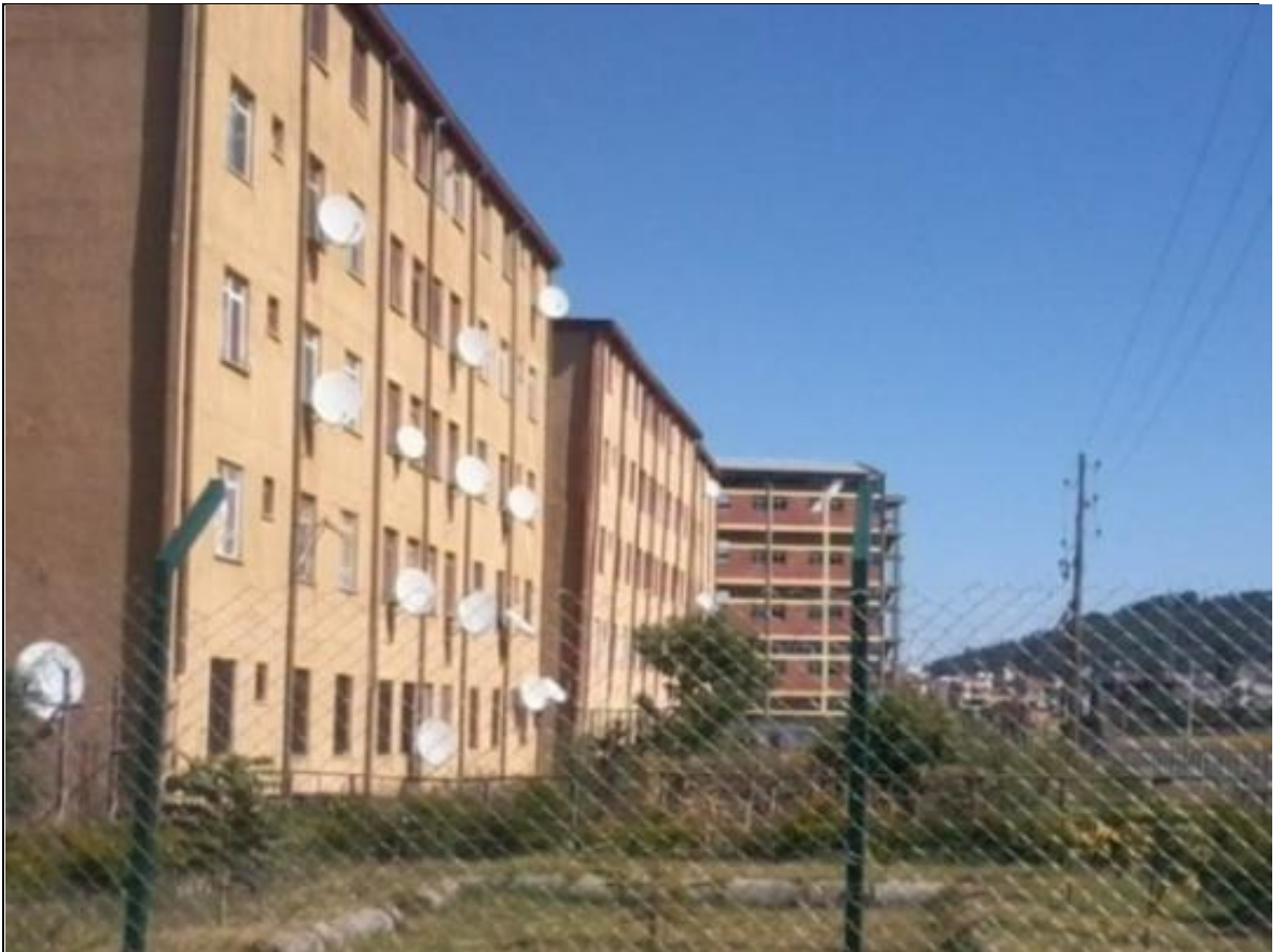
Plate 1.2 Jemo condominium buildings
