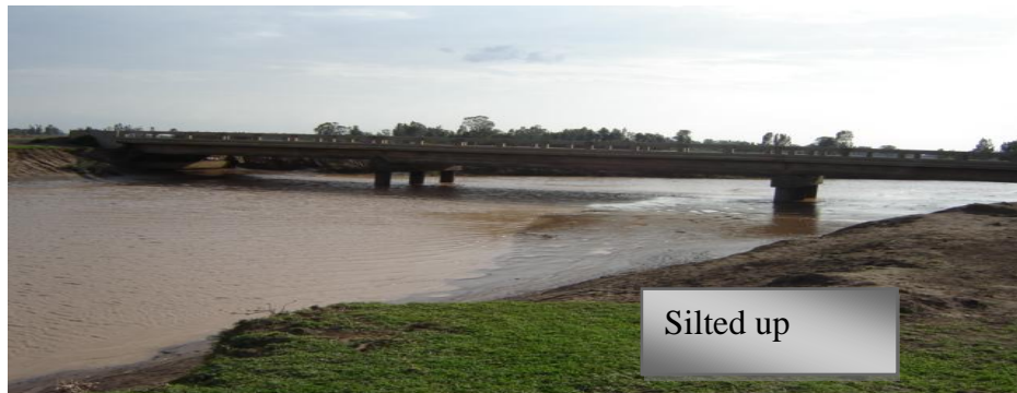
Figure 9: Addis Zemen Bridge at Ribb River (source: MOWE)
