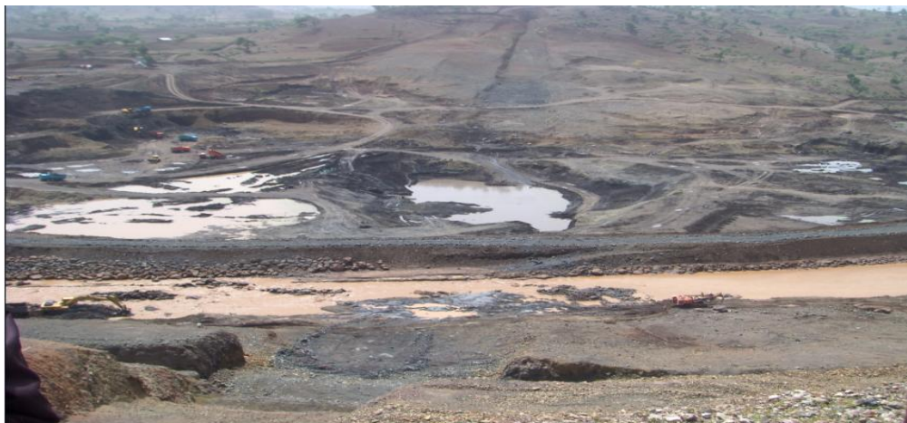
Figure .6: dam site (source site visit)
