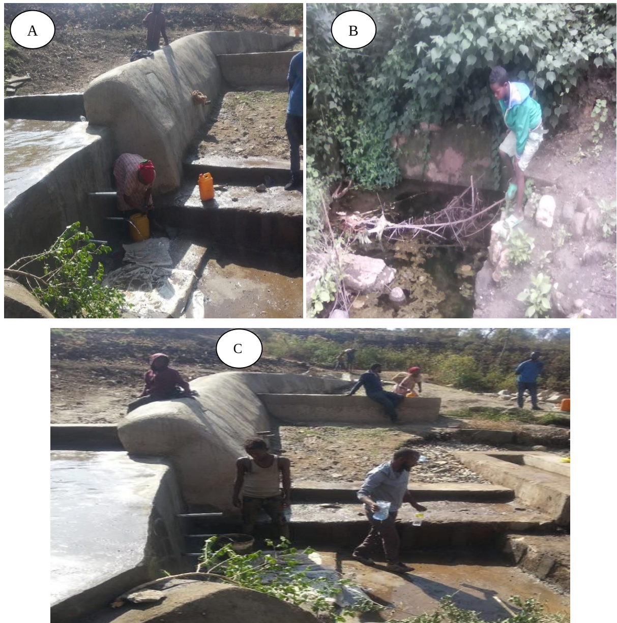
Figure 5. 6 A) and C) developed spring around Sebale kebele and B) Unprotected spring around Kolu kebele
