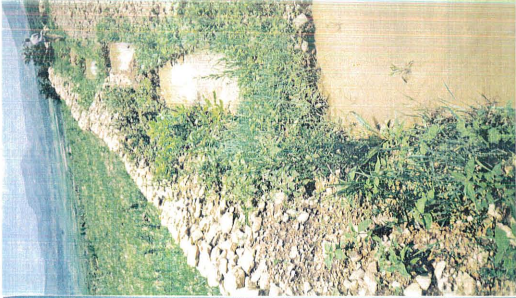
Photo 10. Trench bund above the Korir earth dam
