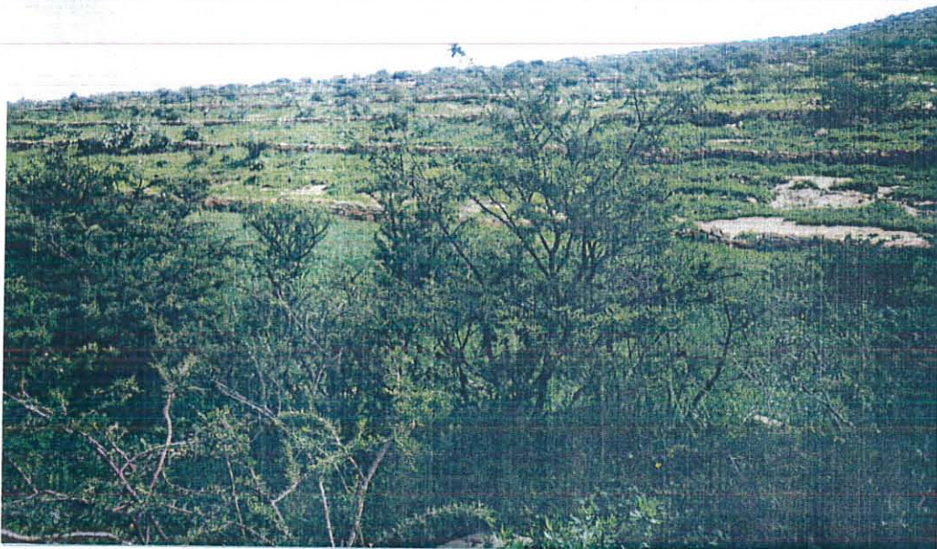
Photo 9. Bund constructed above the Korir earth dam
