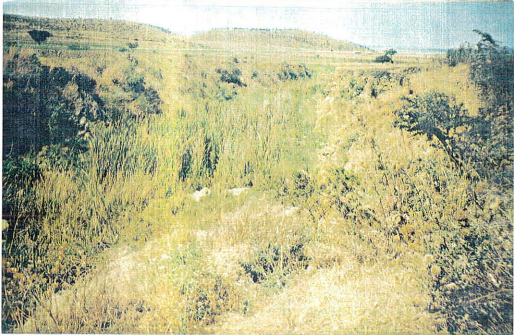
Photo 12. Rehabilitated gully part, below the Korir earth dam
