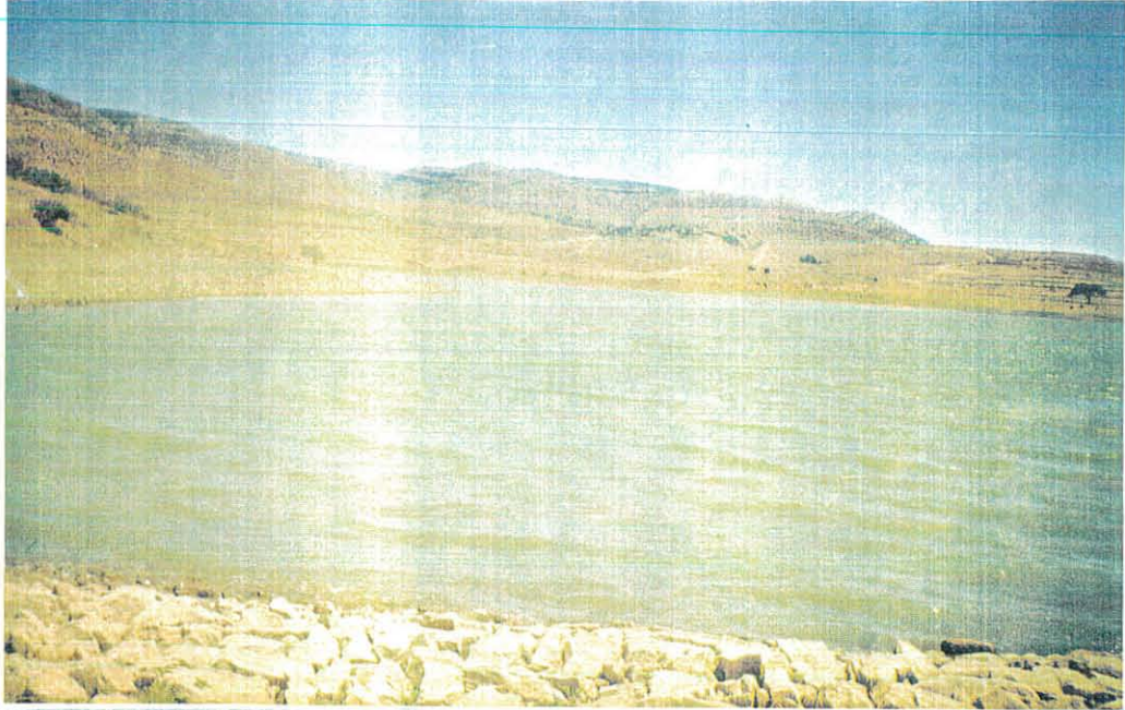
Photo 11. Part of the Korir earth dam
