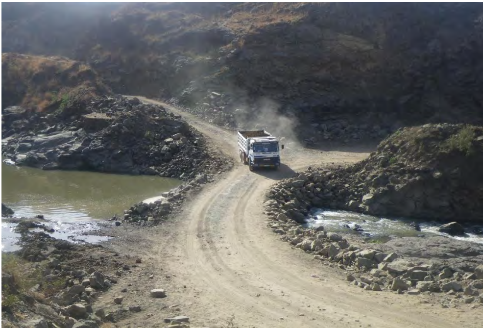
Figure 7: The current access road block the flow of water
