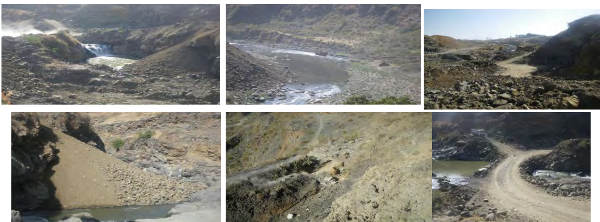
Figure12: Carelessly dumped overburden material and bridging of the river
