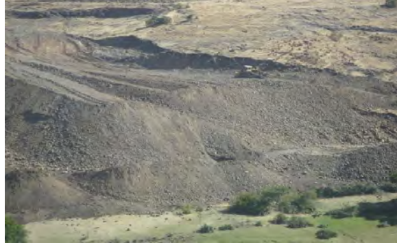
Figure 8: The stripping of overburden material in the study area
