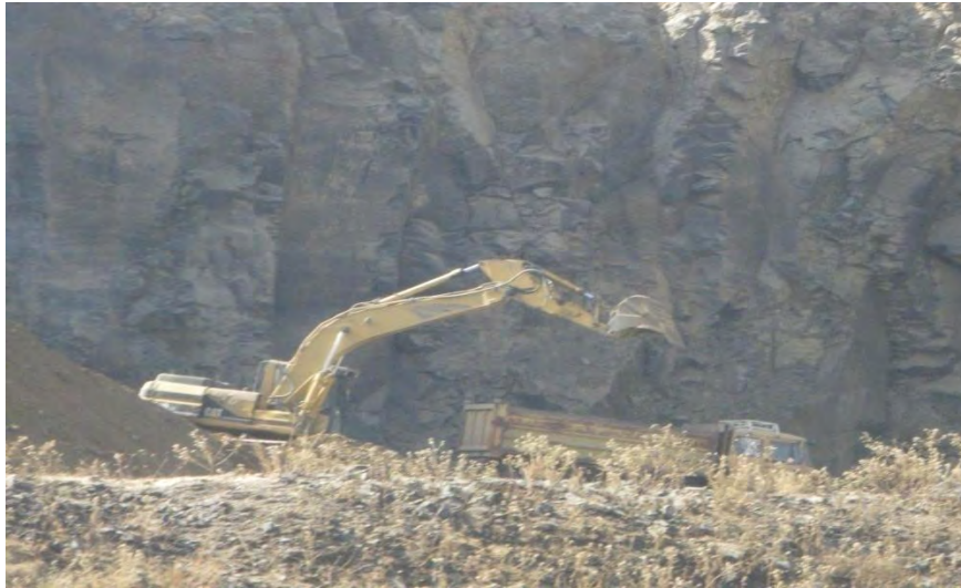
Figure 10: Excavation and loading selected materials in the study area
