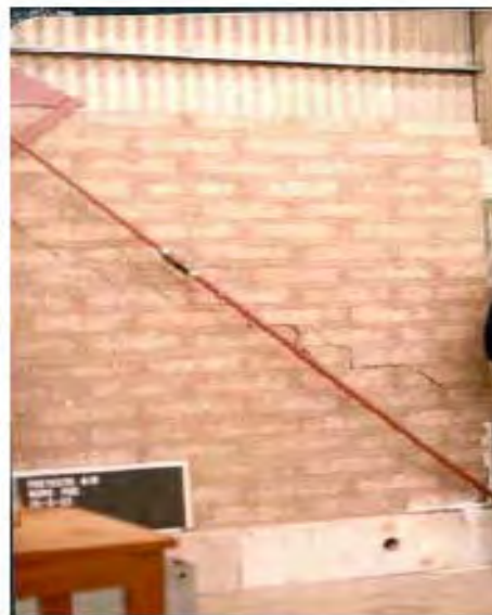
Fig. 4.2.4.4 Full-scale wall test. (Research in Peru 2002)
