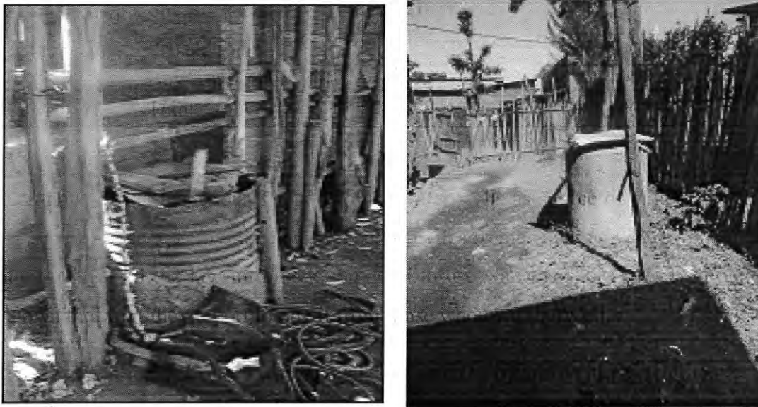
Pic.5.3: Active water Wells at Leku (Left) and Wukro (Right)
