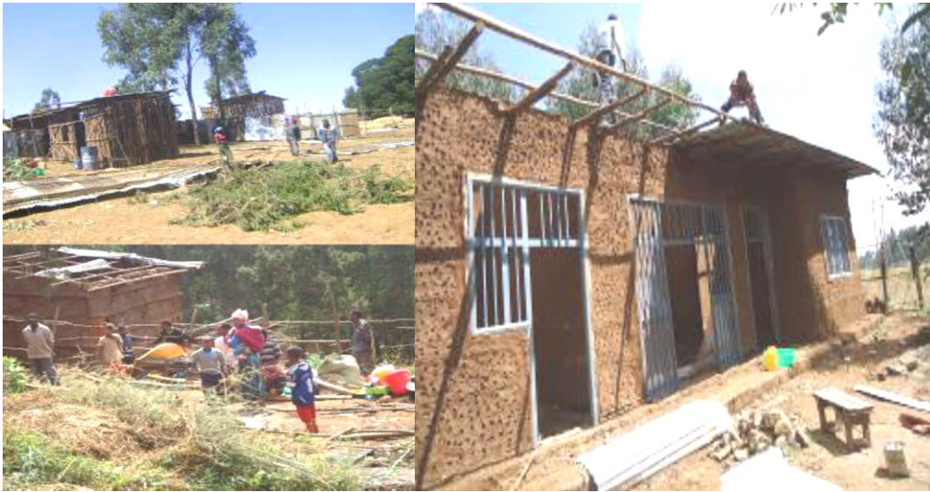
Figure 4. 4: Demolishing operation in Burayu City
