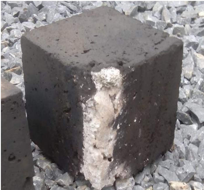
Fig.3.10- Excessive burning caused cement paste bond to spall of.
