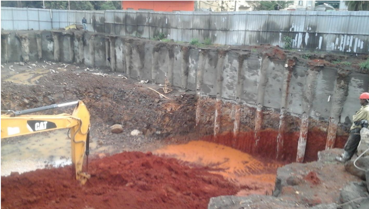
Figure 2.1: contiguous bored pile wall.
