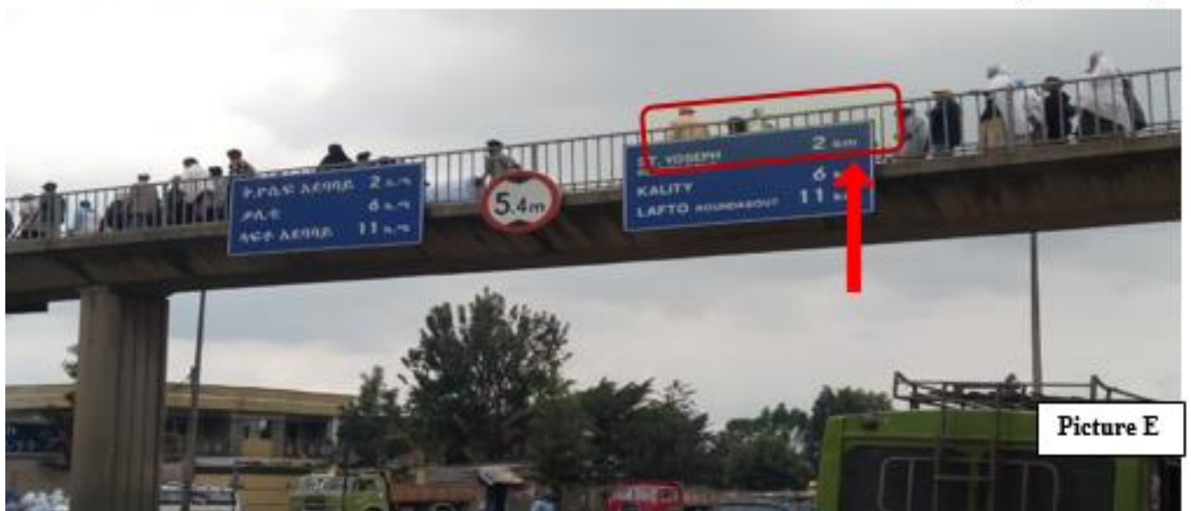
Figure 1.1: Pictures to Exhibit the Problem along the Study Route (Addis Ababa Ring Road)
