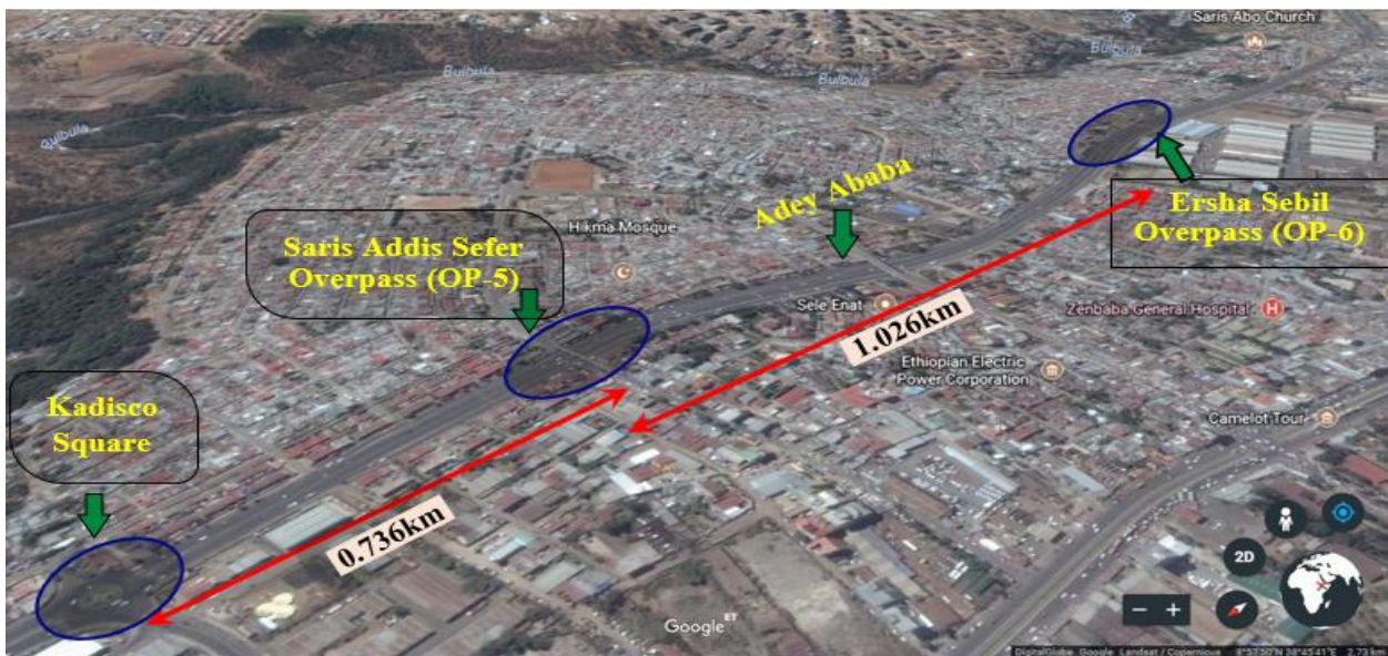
Figure 4.14: Location of Saris Addisu Sefer Overpass (OP-5)
