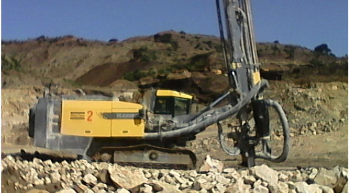
Figure 3-7: Drilling pattern of the quarry site
