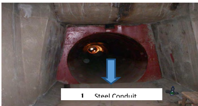
Figure 1-1: View from upstream intersection of conduit with intake foundation
