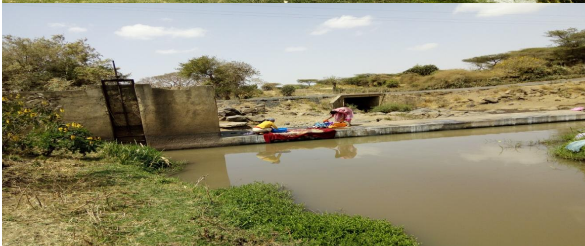
Appendix B- 1: Water Abstraction by Diversion and Pumping at Upstream
