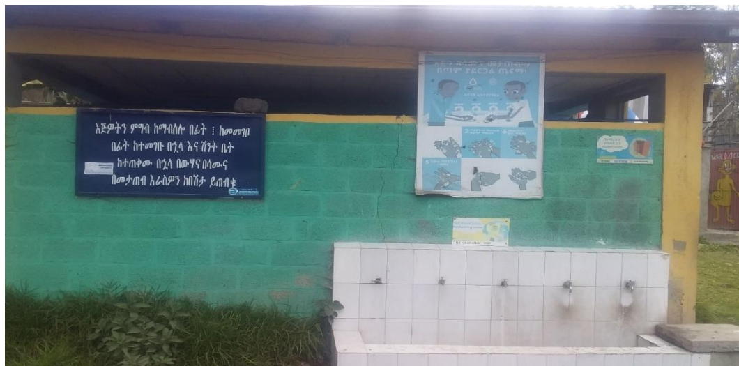
Fig 10. Students' Latrine Room Furi primary School.
