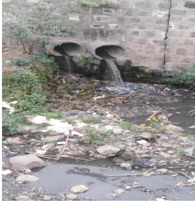
Figure 1-1: Kebena River around Kebena Bridge (18/07/2011 E.C))
