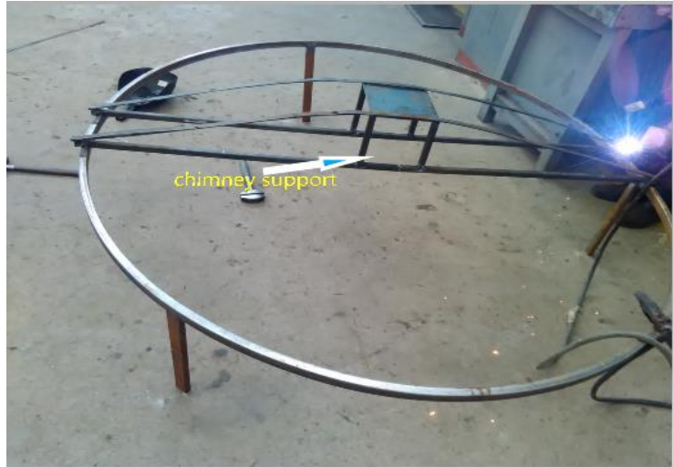
Figure 4-11: chimney load support structure construction
