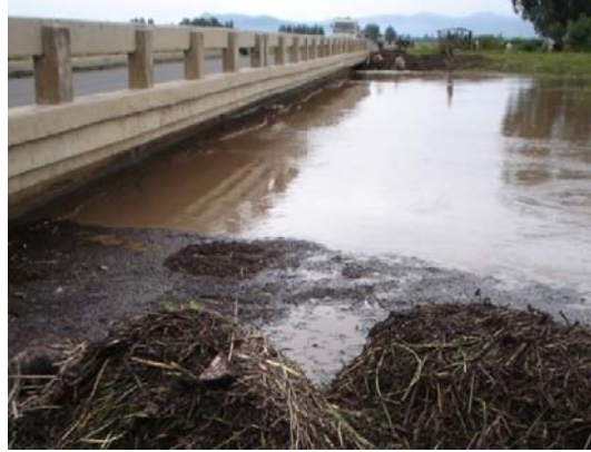
Plate 3.2: Gumara Bridge (Along Bahir Dar to Woreta)
