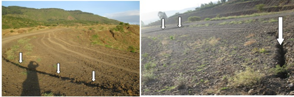
Figure 1. 2 Cracks across the road
