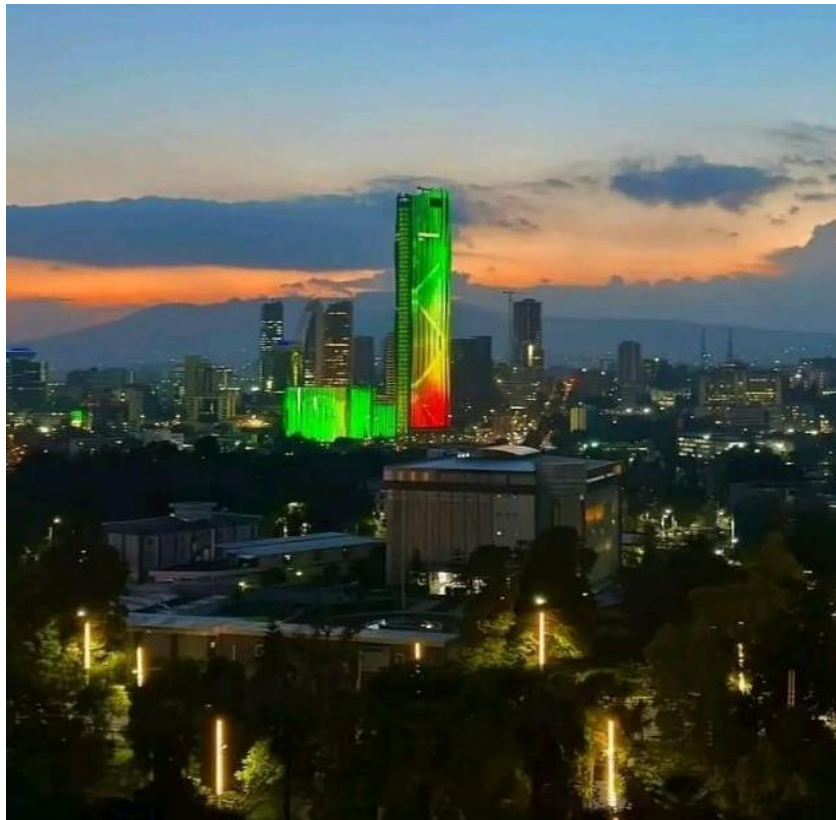
Figure 1-2: CBE new headquarter building
