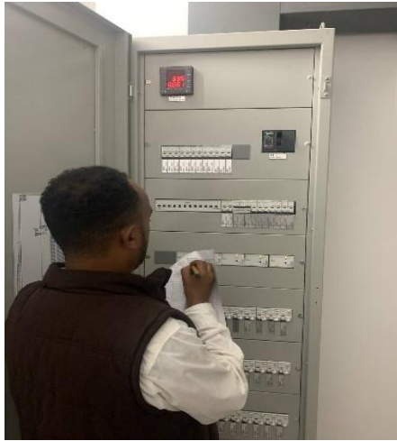
Figure 7-9: Lighting energy consumption reading recording procedure
