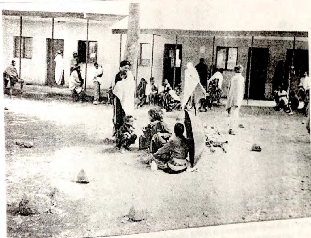
Figure 4. This is a photograph of Jawi health center
