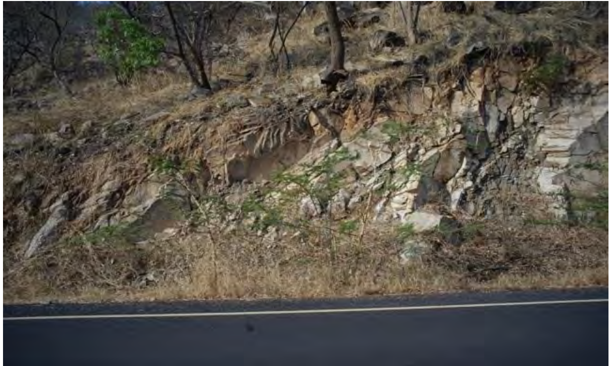
Plate 6.2. RMR point 8, left side of the outcrop left abutment
