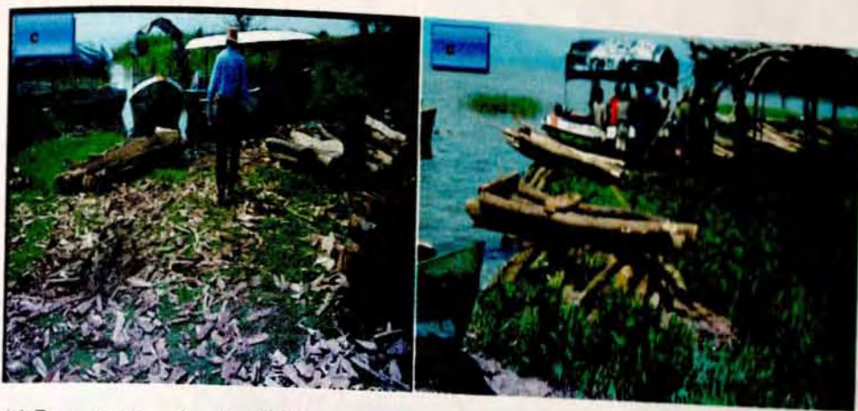
(c) Boat construction for fishing and associated plant species loss ( Aeschynomene elaphroxylon ) in Lake Abaya and Chamo
