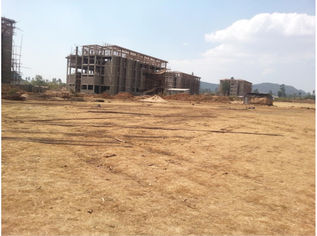
Figure 1.2. Partial view of the construction site
