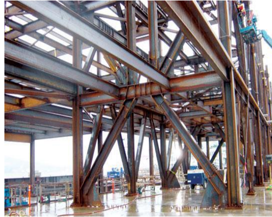
Figure 2.6: Eccentric Bracings
