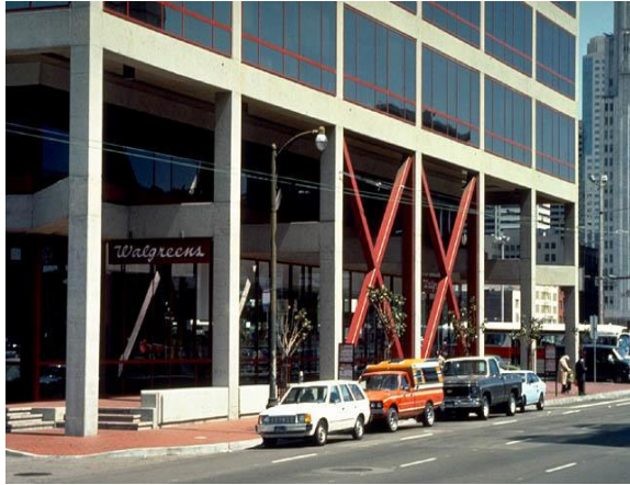
Figure 2.5: Concentric Bracings
