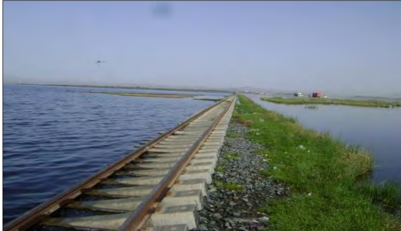
Fig.3.4.2e. Submerged railway access (OWWDSE2014)
