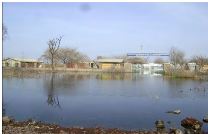
Fig.3.4.2d. Submerged public health center (OWWDSE 2014)
