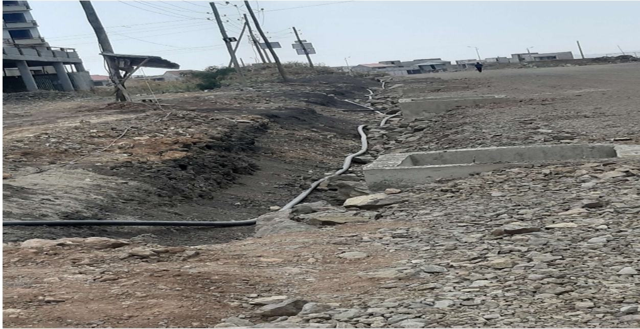
Figure 5: The existing water supply line in the project site/field observation.
