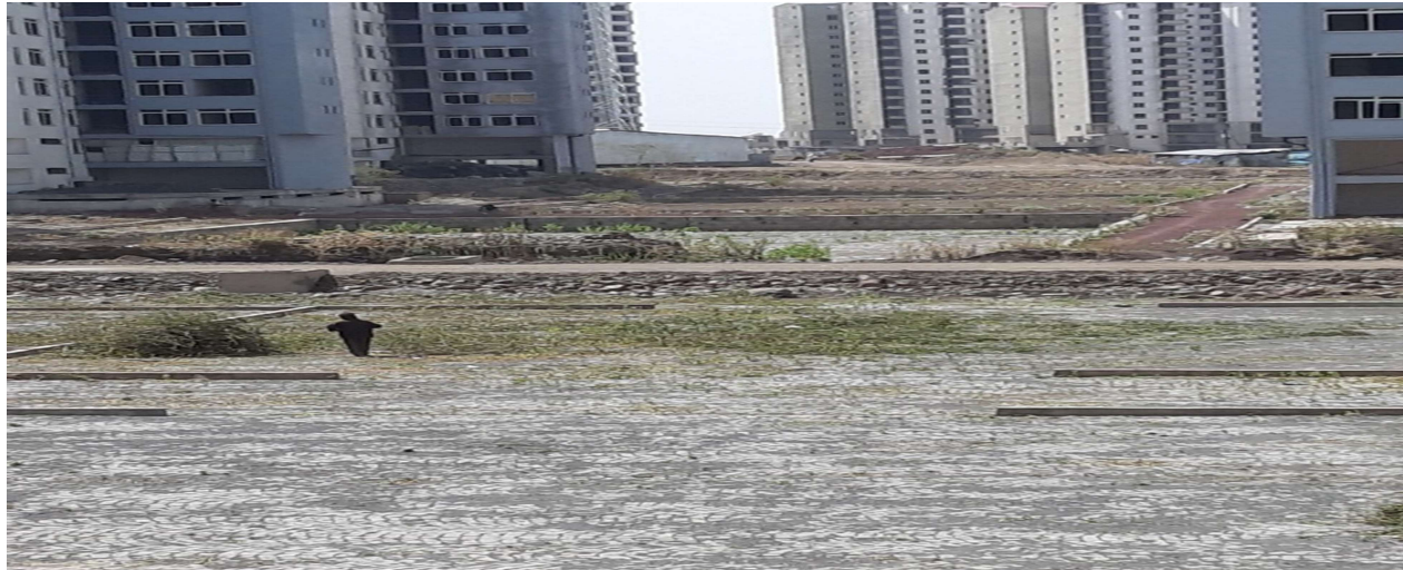
Figure 6: A figure showing the elevation difference of the two car parking's/field observation.
