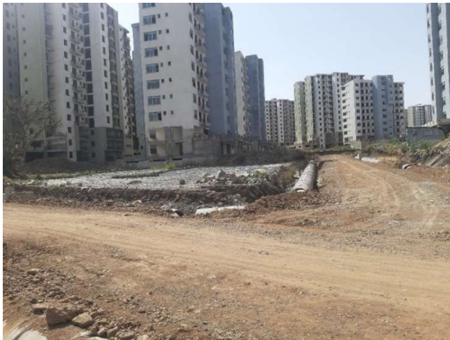
Figure 9: A figure showing the demolished sides of a car parking. As an expert from the target institutions revealed, the car parking in the above figure was constructed before the beginning of the main road between the blocks in the project site. This had caused to demolish part of the already constructed car parking (the two sides of the car parking) to accommodate the design of the road width. As another expert from the same
