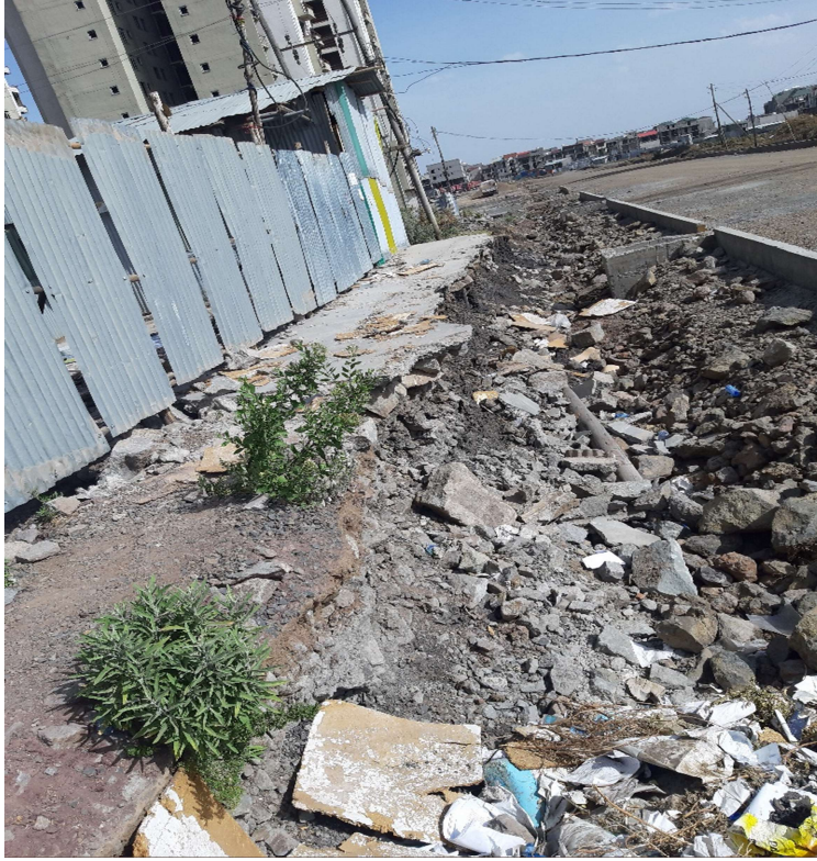
Figure 7: A figure showing a partially demolished project office/field observation.
