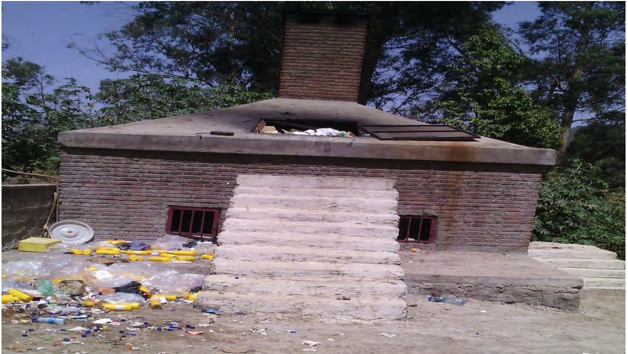
Figure 9: A newly built incinerator for HCW incineration of Menellik II Hospital, February 2015.
