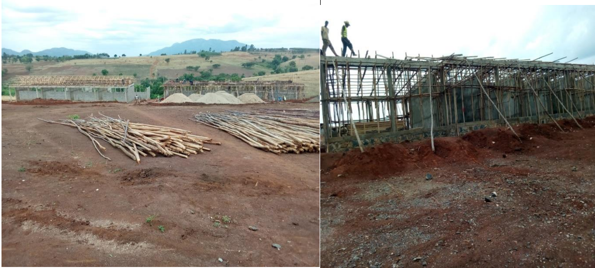
Picture.7.1 Inclusive secondary and preparatory school under construction taken by researcher on 22/05/2019
