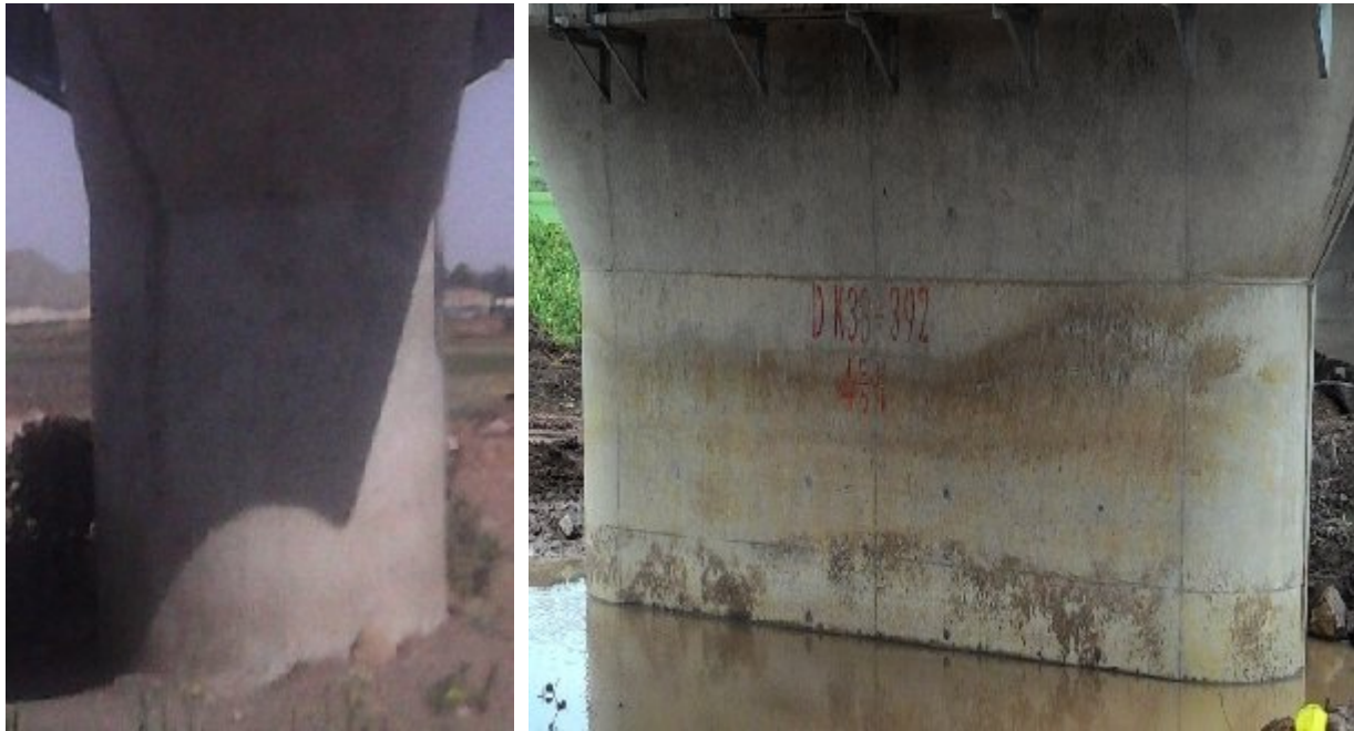
Photo 4-2: Akaki New railway Bridge Pier shape
