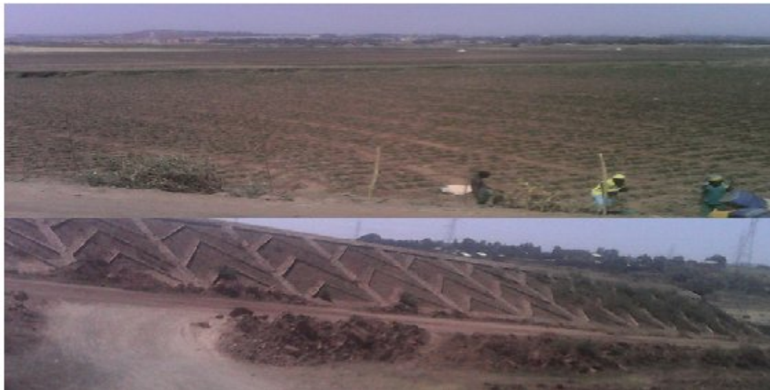
Photo 1-1-2: Flood plain and Embankment at Akaki new railway crossing (Jan 2014)
