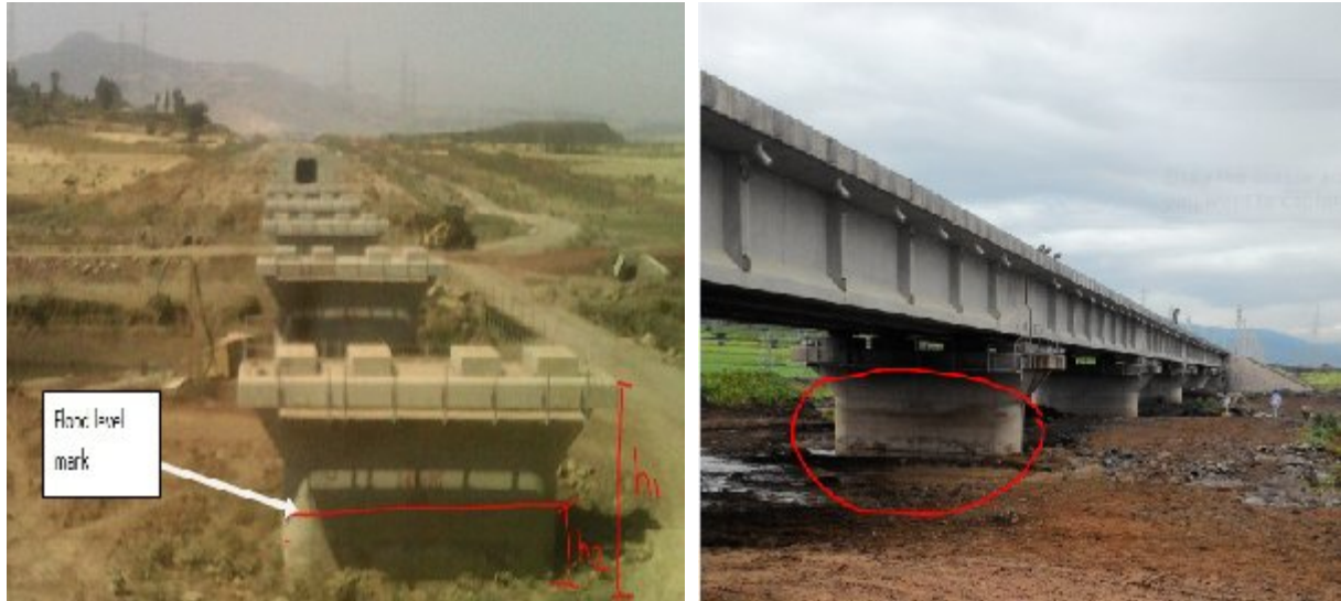
Photo 1-1-1: Flood level mark on Akaki River crossing Railway Bridge
