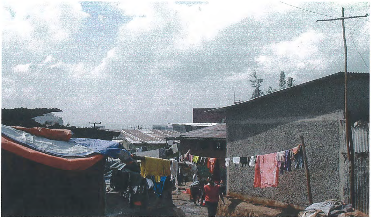
Figure 3.8: The Source of Electricity for Informal Settlers Source: Field survey 2010
