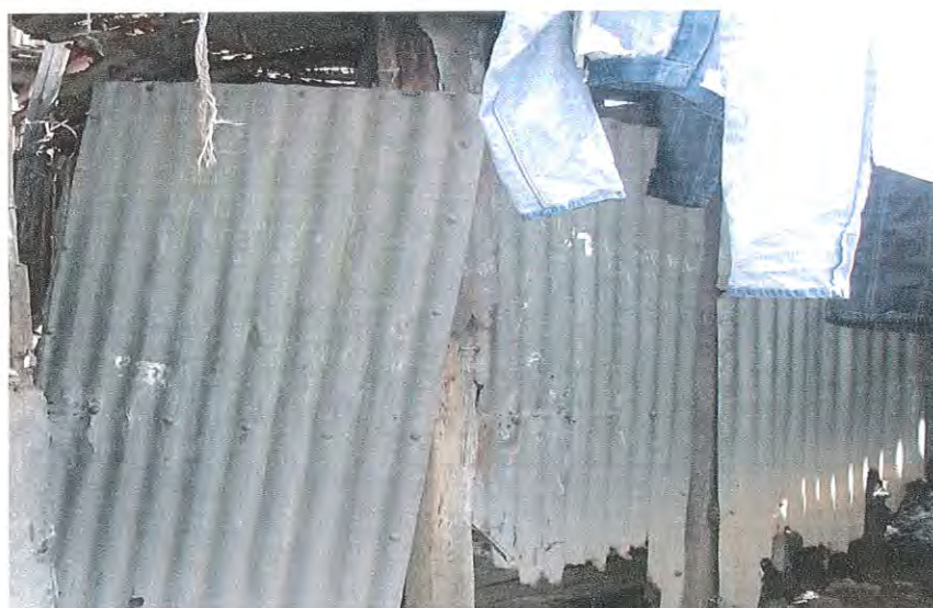
Figure 3. 6: The Condition of Communally Used Toilet Rooms Source: Field survey around, 2010
