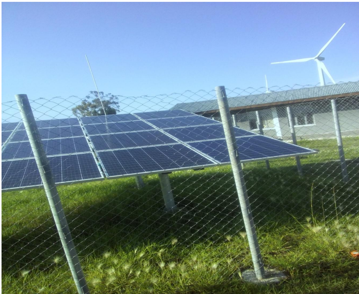
Fig.25.Solar panel 4050 watt that used as source of power for Mukoye Haro health station
