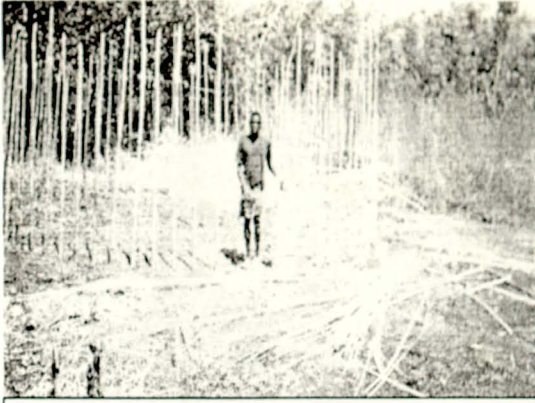
Plate 19: A house on construction
