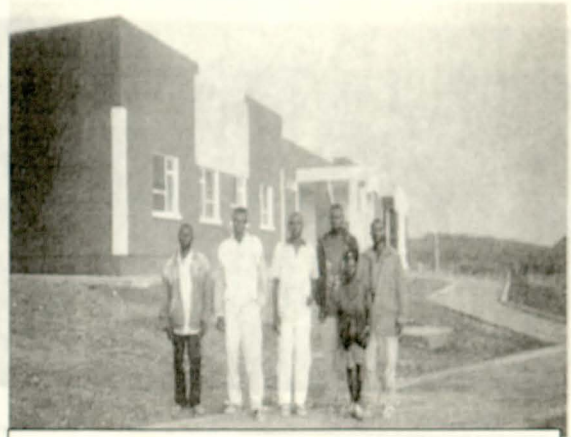
Plate 8: A view of zone council's building from right
