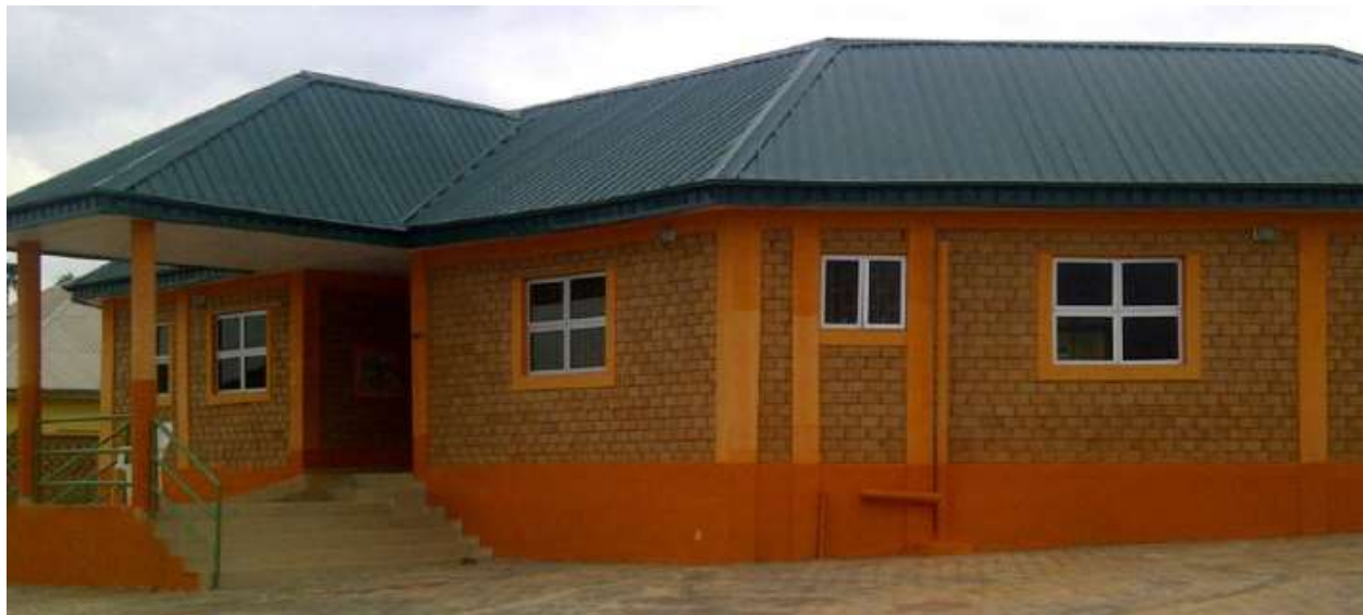
Figure 2-9: CSIEB used for the construction of a caring heart mega school, Ondo state, Nigeria
