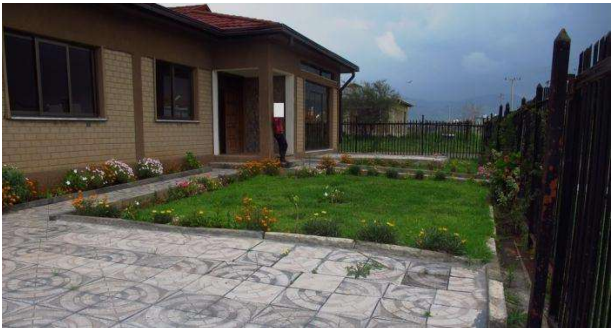
Figure 2-13: villa house in Ropack real estate, wall built with CSSBs. Lage T’afu, Ethiopia
