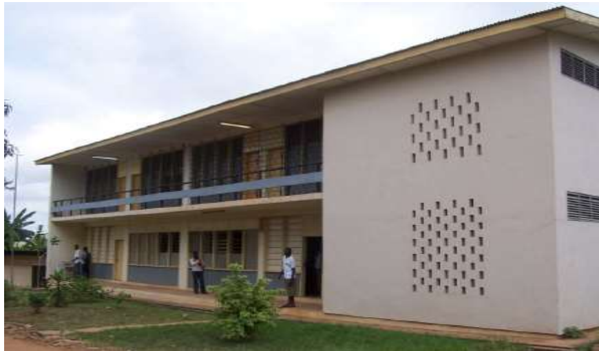
Figure 2-10: Two-storey Office Block for DHPR on Kwame Nkrumah University Science and Technology (KNUST) campus built with CSSBs
