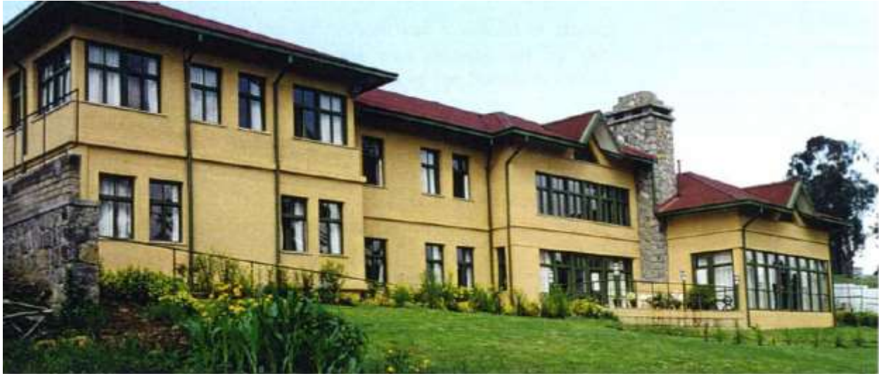
Figure 2-12 Save the children, Office building, Addis Ababa [6]
