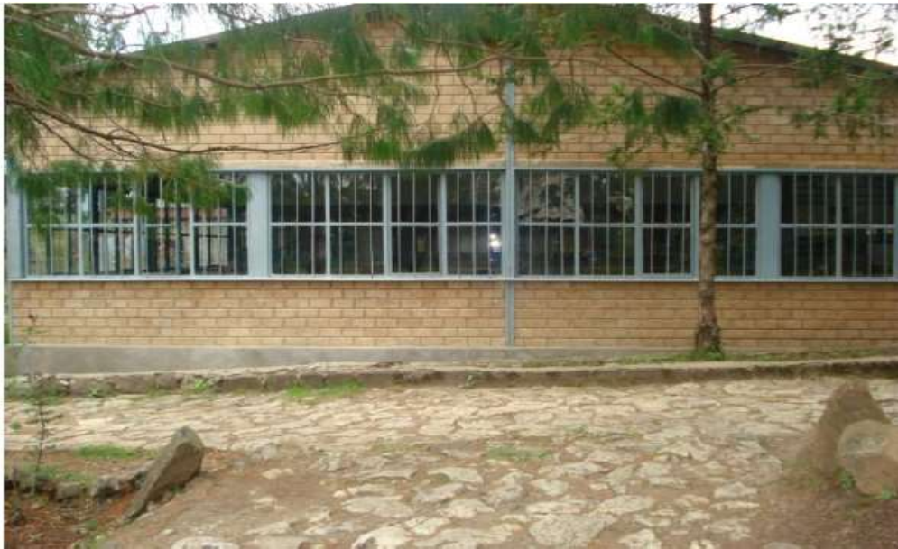
Figure 2-11 The kitchen facility at STVC, built with interlocking CSSB [6].
