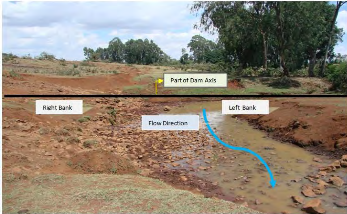
Plate - 6.3 Portion of Alluvial Soil Foundation at the left valley floor area
