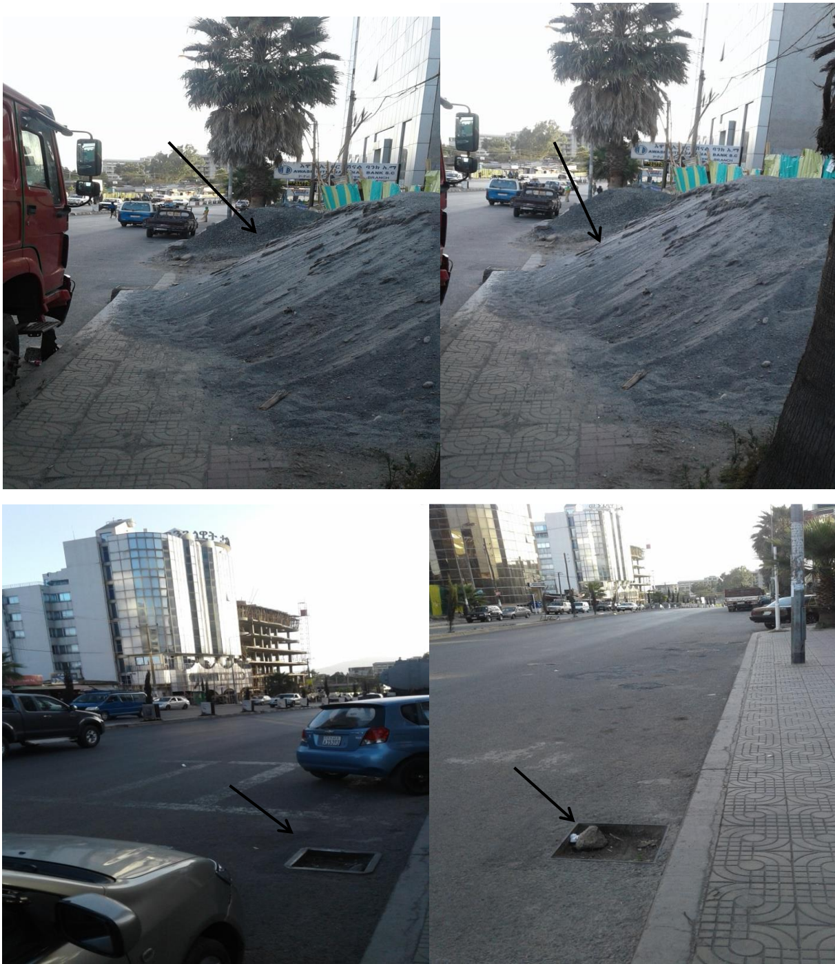
Figure 16. Photo. Construction materials dumped on the walkway, blocked ditches
