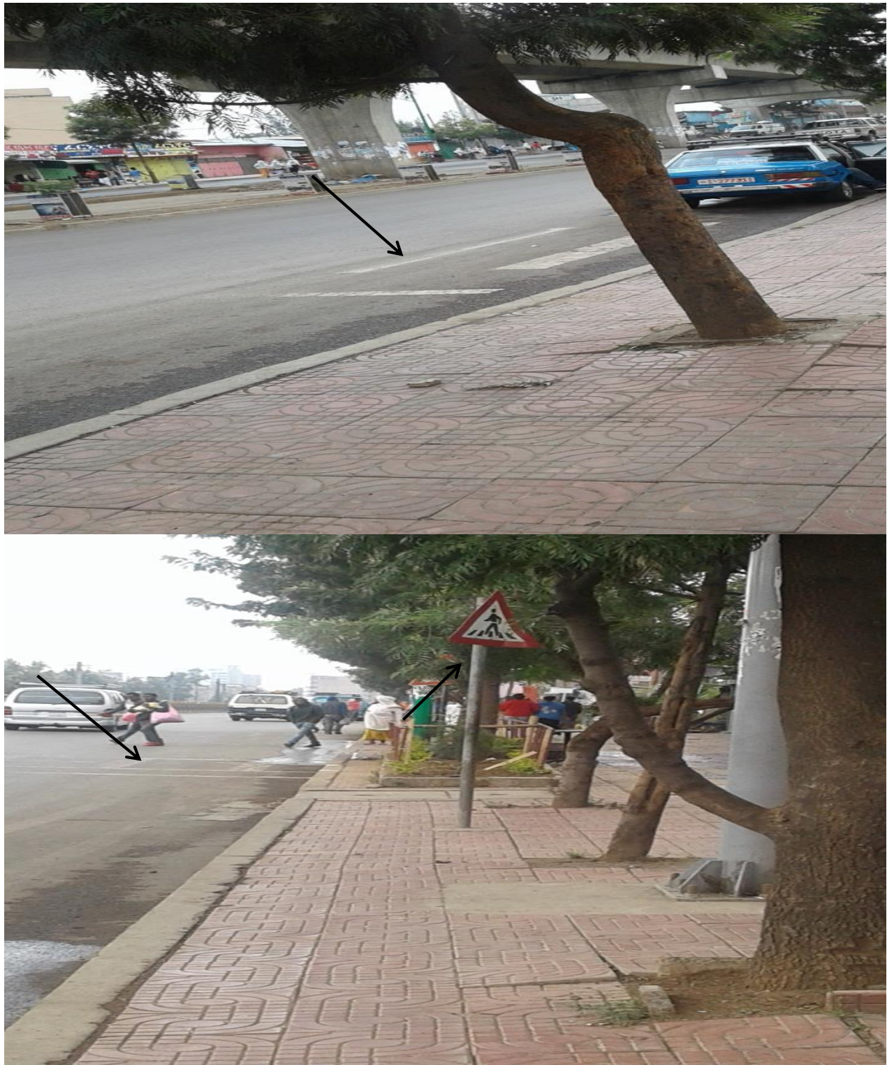
Figure 41. Photo. Faded pedestrian cross marking, damaged traffic sign, Long Branch of road side trees.
