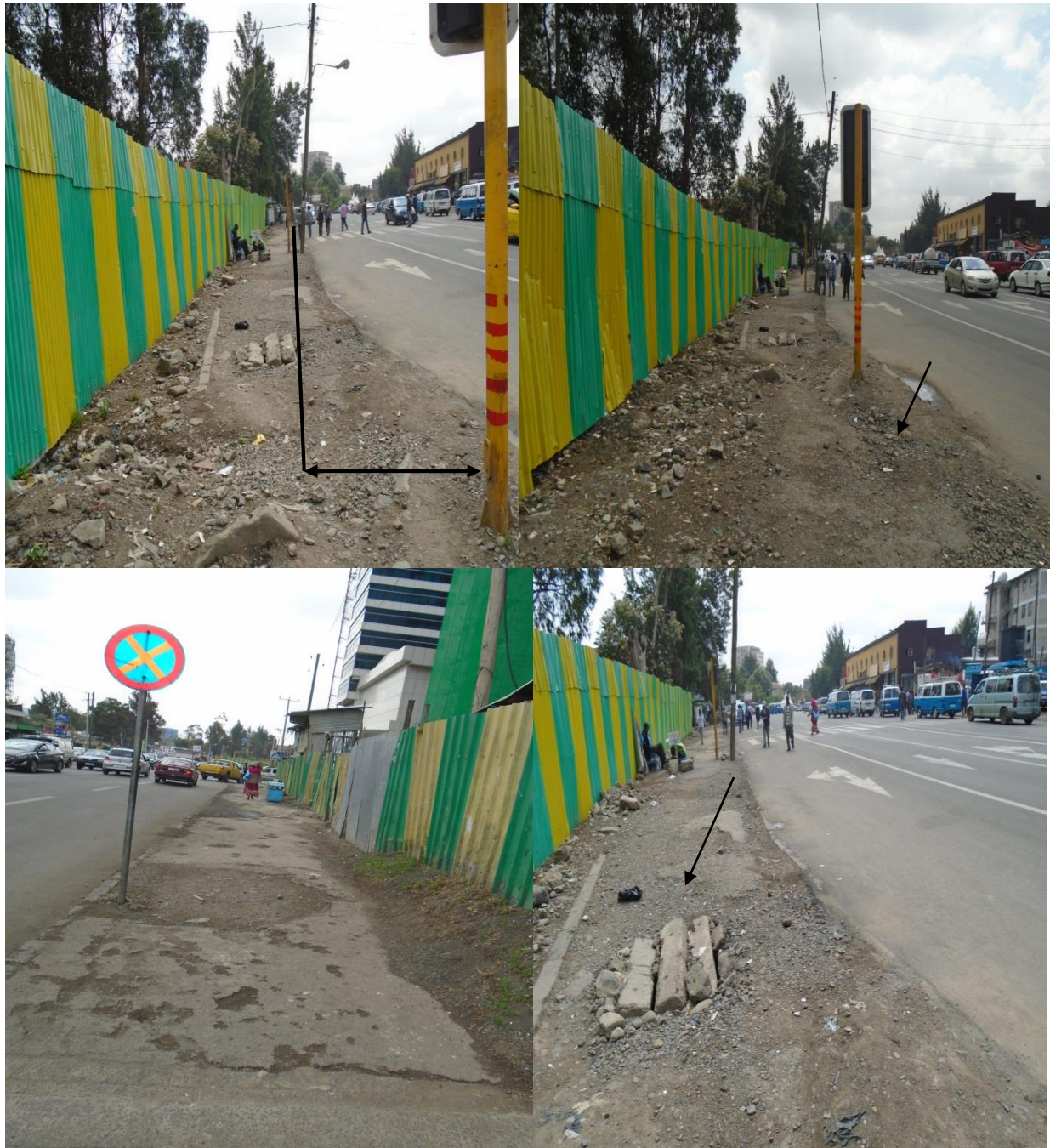
Figure 3. Photo. Signals at the wrong position and are not functional, missing kerb, surface defect of walk way
