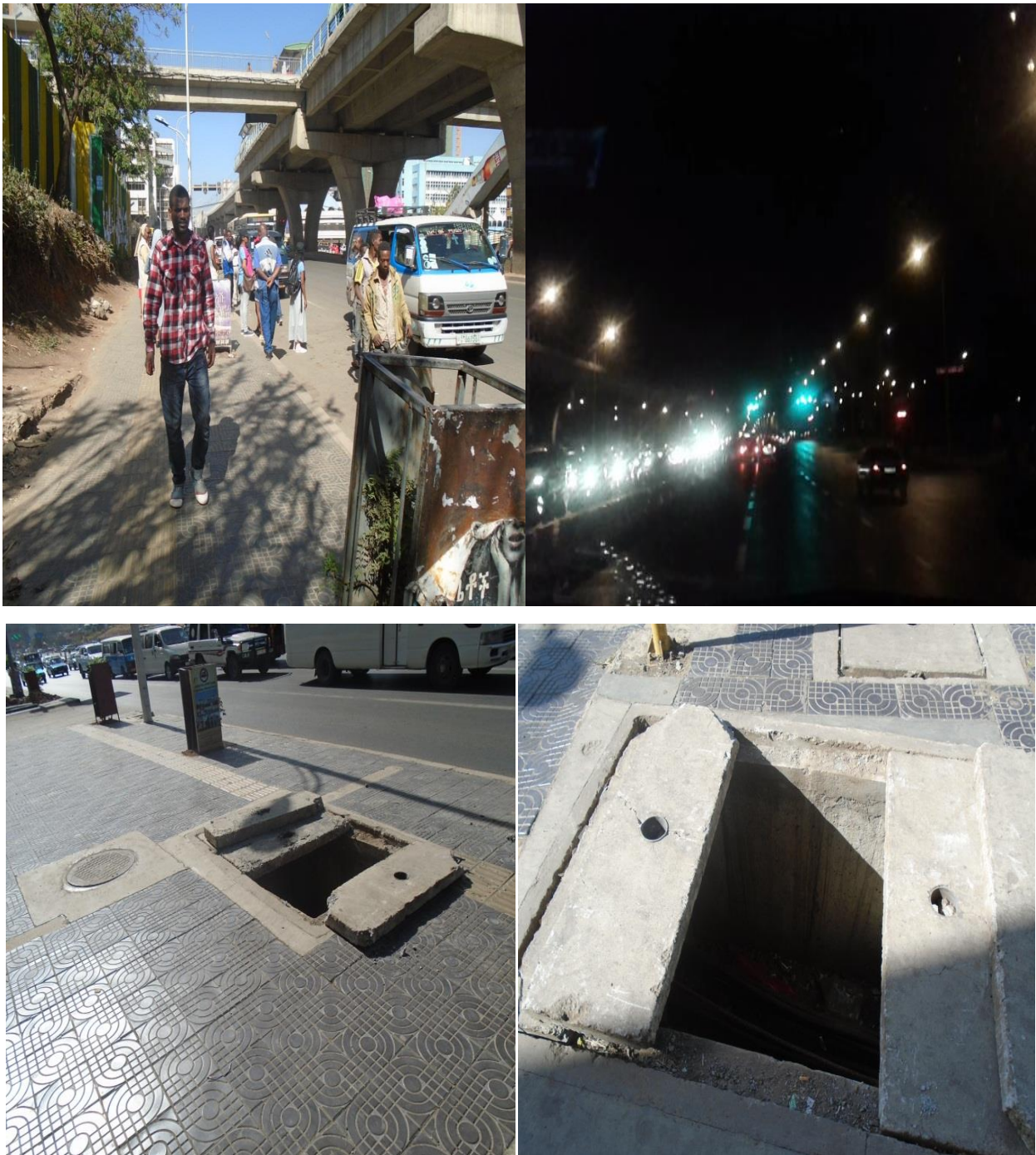
Figure 8.Photo. Insufficient passenger facility, good visibility of road marking and lighting, unprotected opened utility line manholes.
