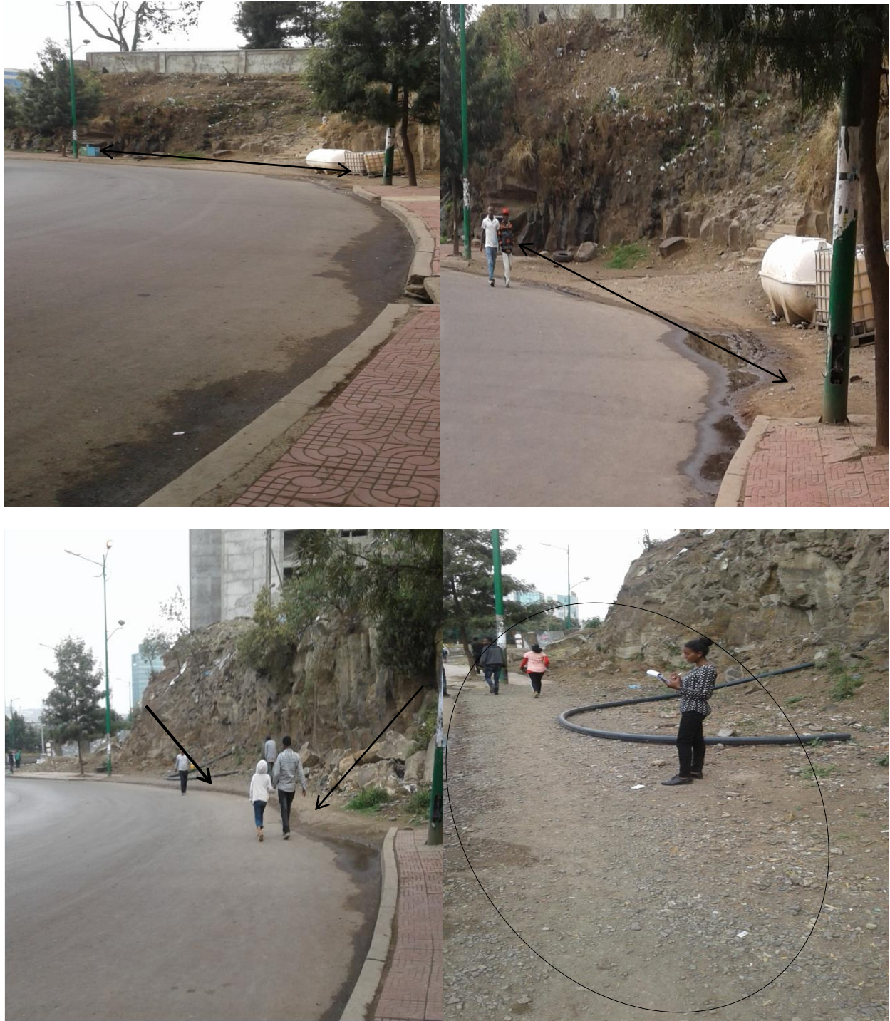
Figure 40. Photo. Provision of pedestrian walkway is not continuous on both sides of the road
