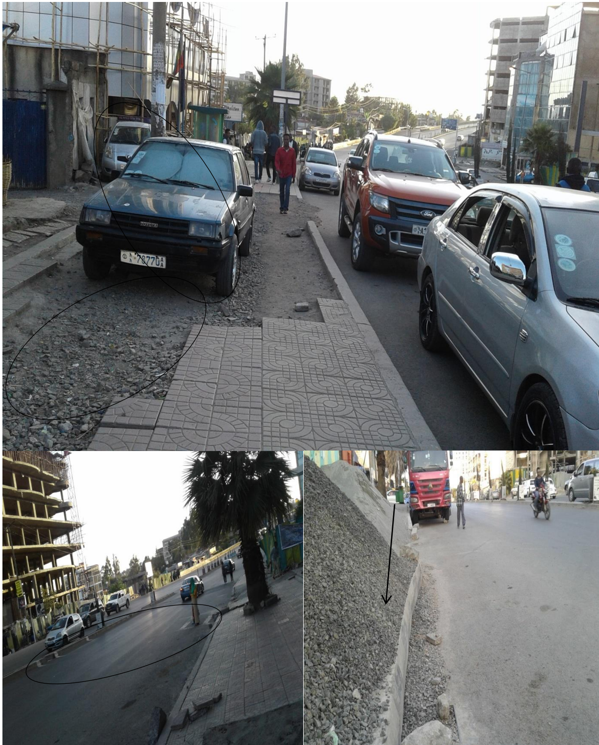
Figure 15. Photo. Damaged walk way, vehicles parked on walkway, faded pedestrian cross marking and dumped construction material on walkway
