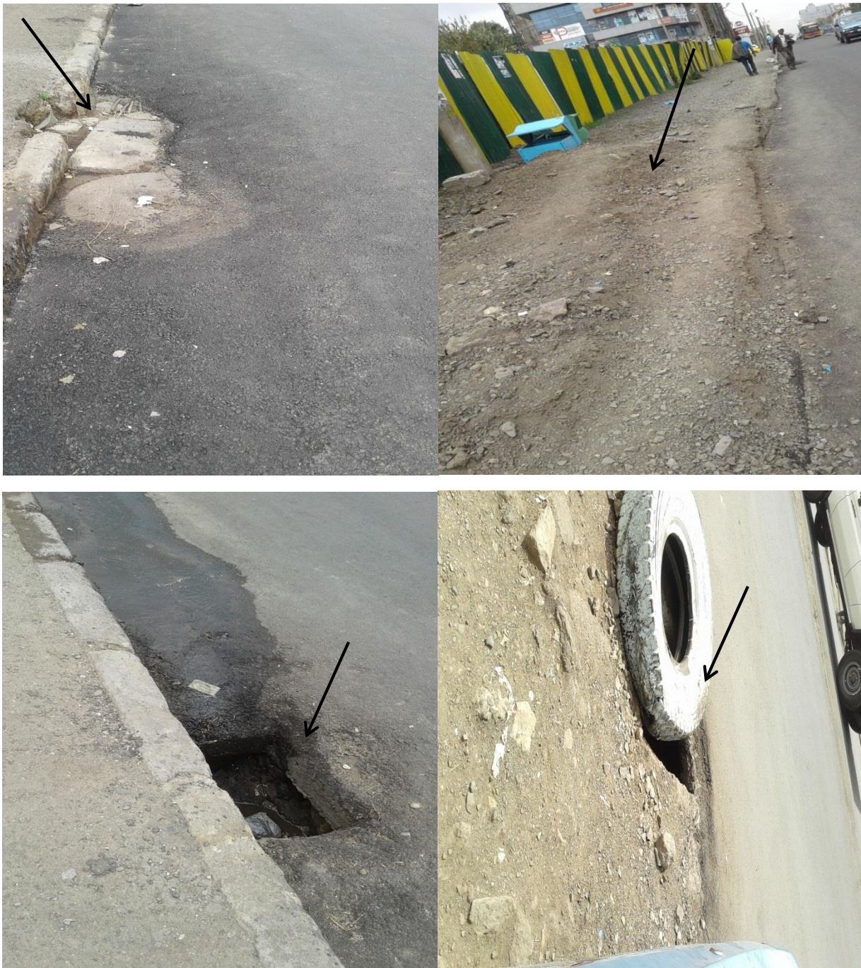
Figure 33. Photo. Blocked road side inlet, construction debris on walkway, uncovered ditch, and improper drainage cover
