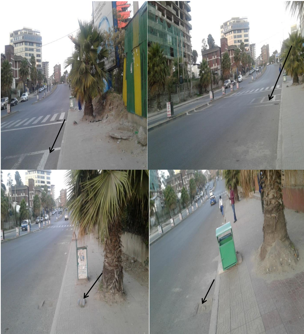
Figure 11. Photo. Old cross marking is not removed, damaged lighting, blocked inlet
