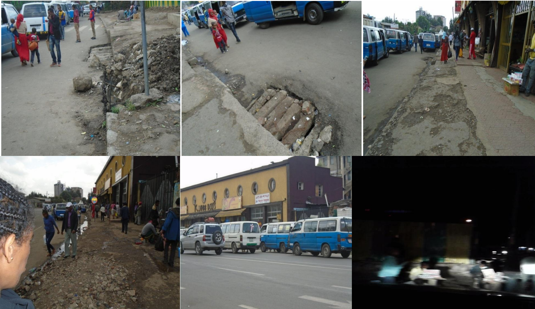
Figure 5. Photo. blocked drains, Insufficient pedestrian and passenger facility, the service area and taxi station very close to each other, worn walk way, insufficient parking space for taxis, road side vendors at night, no road side lighting.
