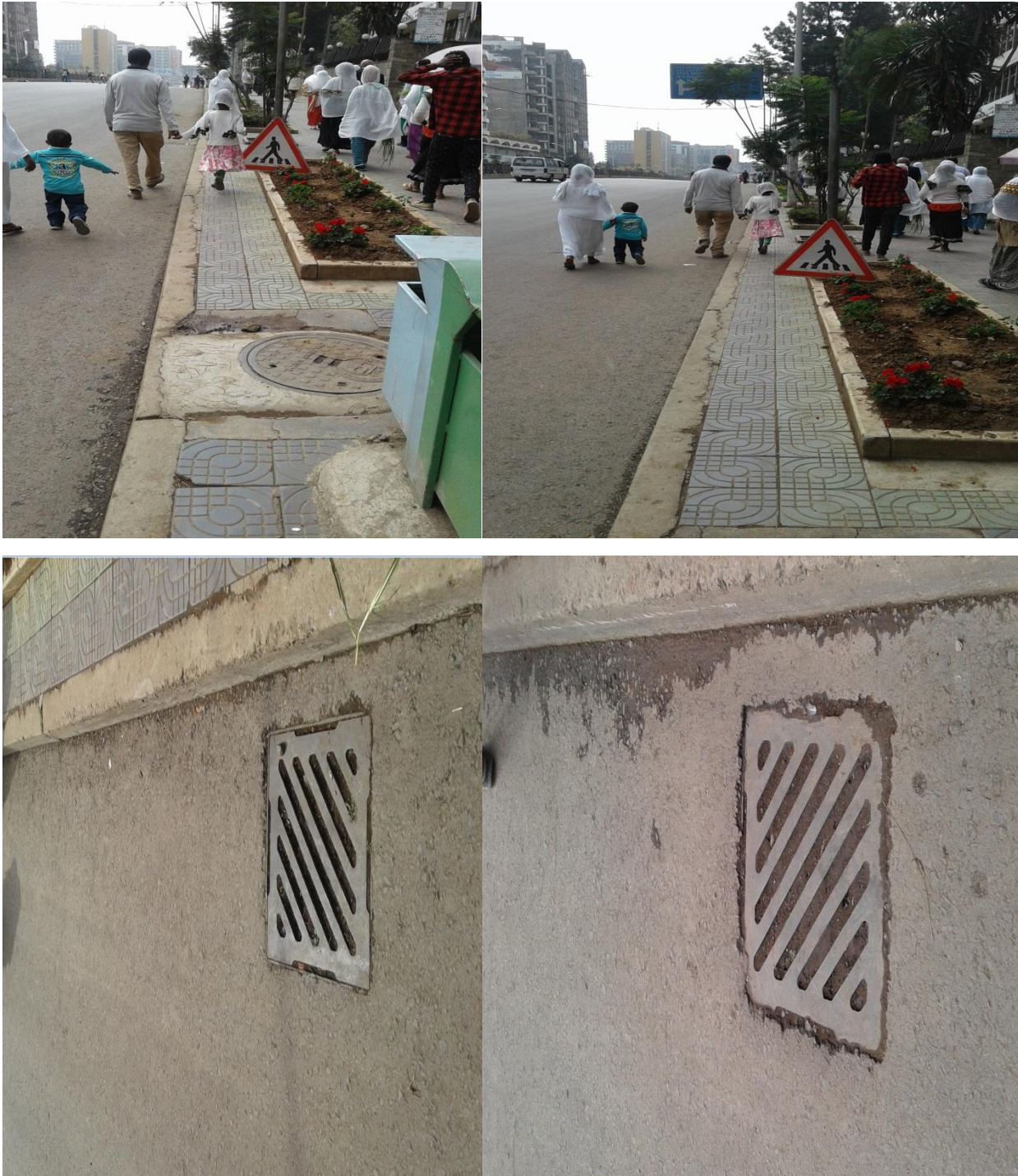
Figure 21. Photo. Damaged traffic sign, blocked inlets
