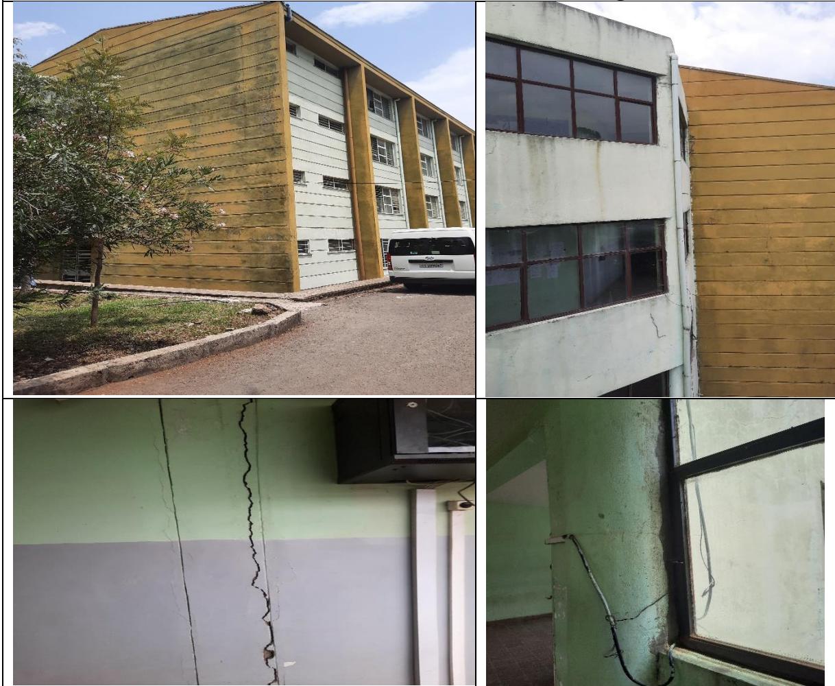
Built Asset Condition
