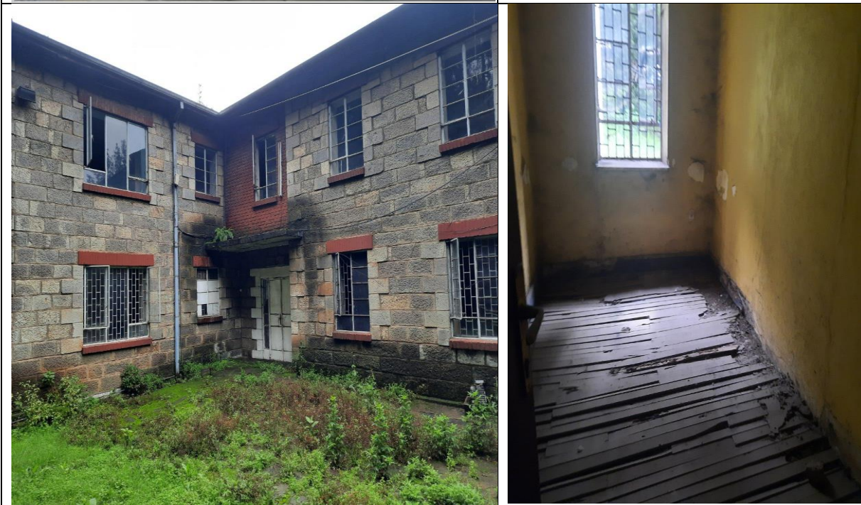
Built Asset Condition
