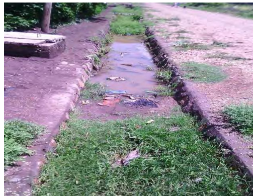
Figure 2-12: Open drainage system with no outlet(Asfaw, 2016)
