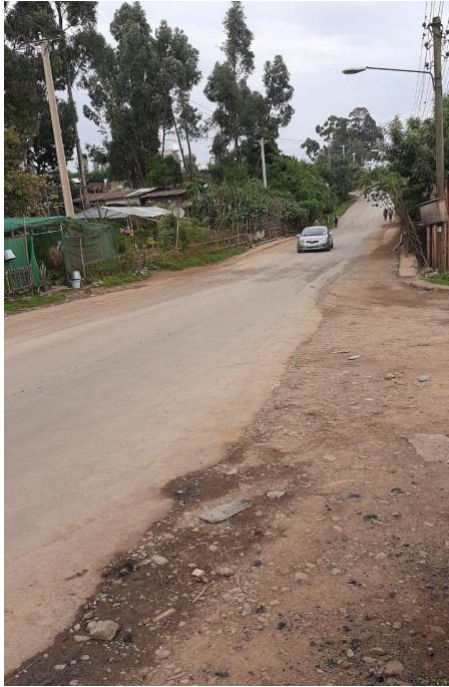
Figure 4-1: Street of Dera Sefer area with a steep slope (Author, 2020)
