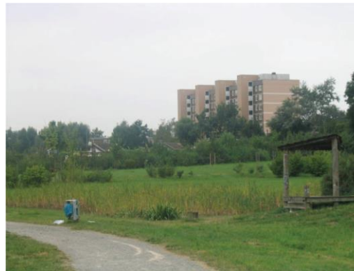
Figure 2-6: GI implemented for stormwater management on the property of public housing in the Emscher region (Nickel et al., 2014)
