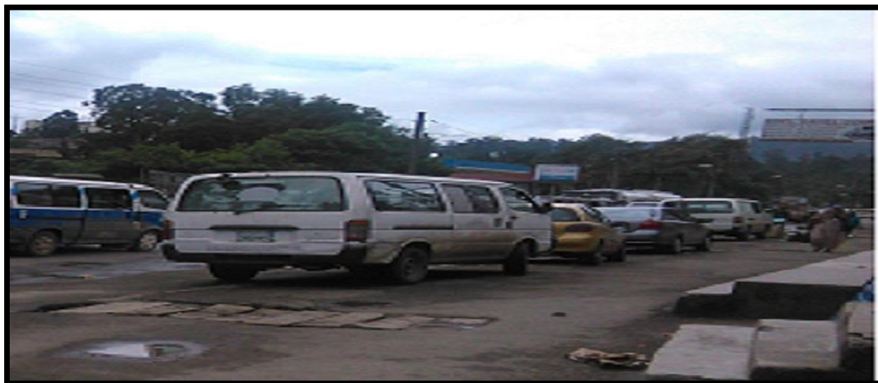
Figure 4.14: Illegal parking on the edge of the road and pedestrian walk way due to narrow road width, R-011 at Yegna guada bar and restaurant
