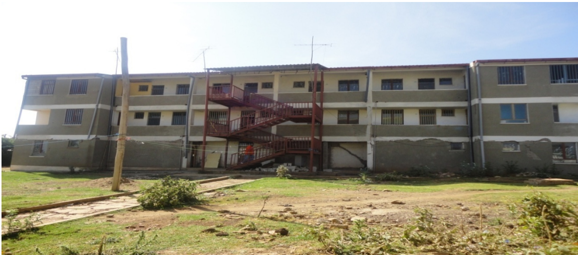
Figure 4.1: Front view of case study 01
