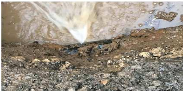
Corrosion pin hole on an iron pipe.
