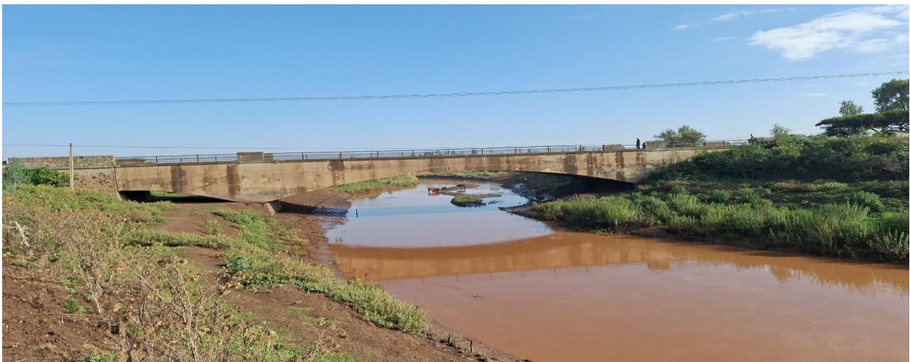
Fig. 28 Awash River bridge at Tefki district
