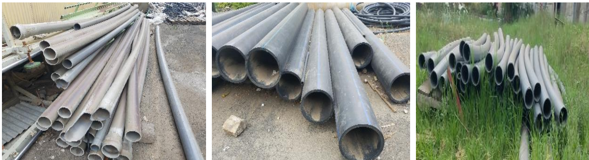
Figure 13: Observed quality defect poor material handling
