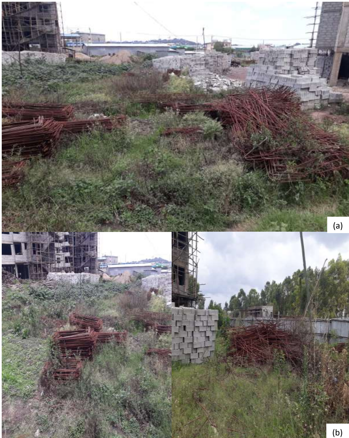
Figure 4.7: Buried Rebar due to delay in client collecting remaining pieces
