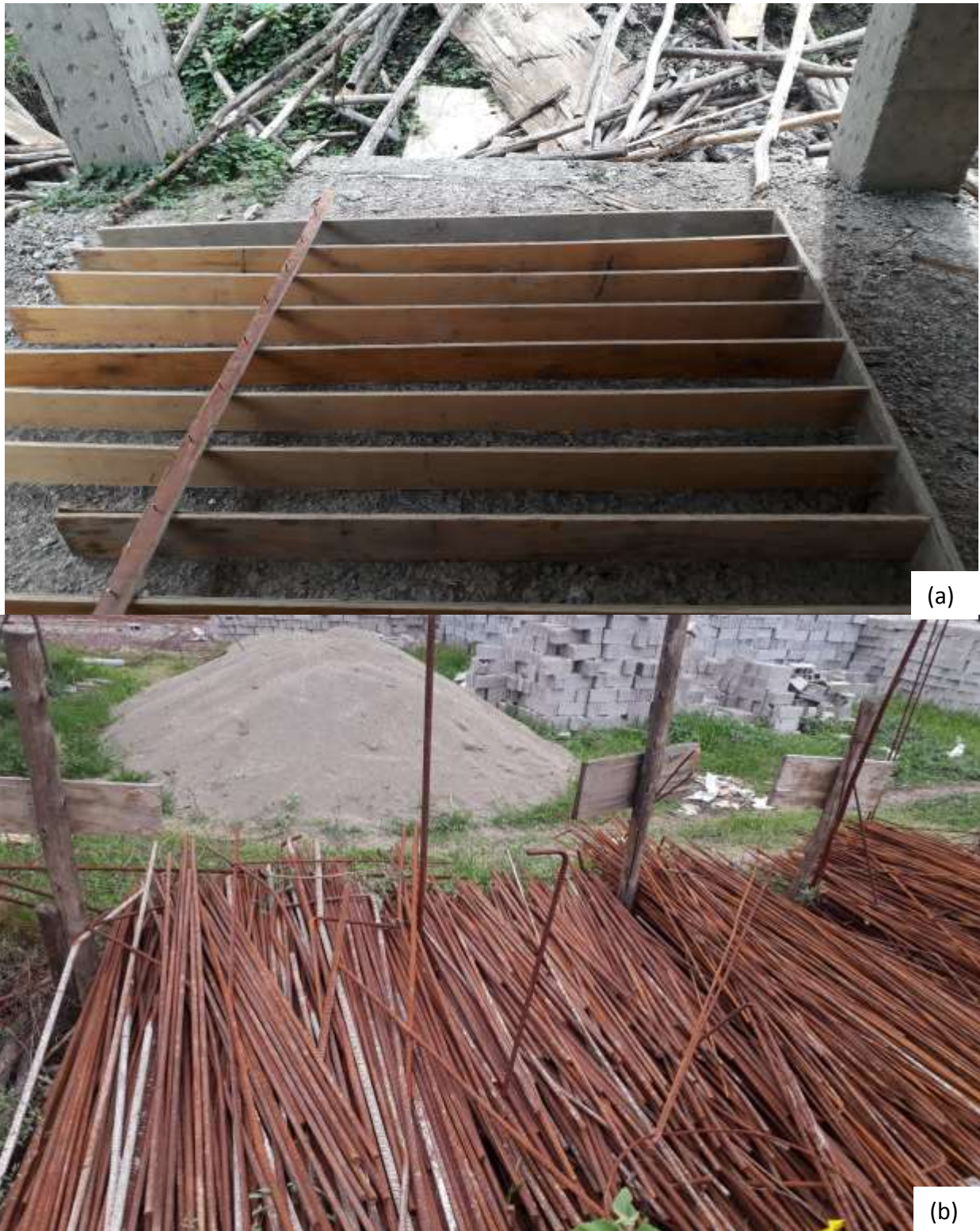
Figure 4.4: Appropriate rebar bed used for arrangement of rebar after cutting
