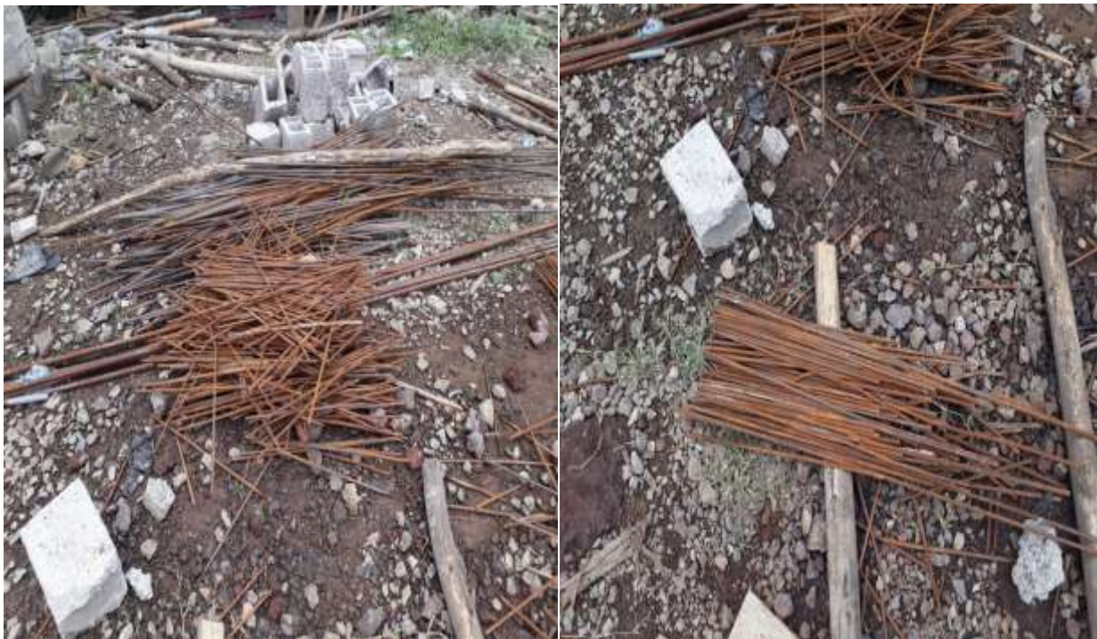
Figure 4.6: Before and after an arrangement of Rebar cutoffs
