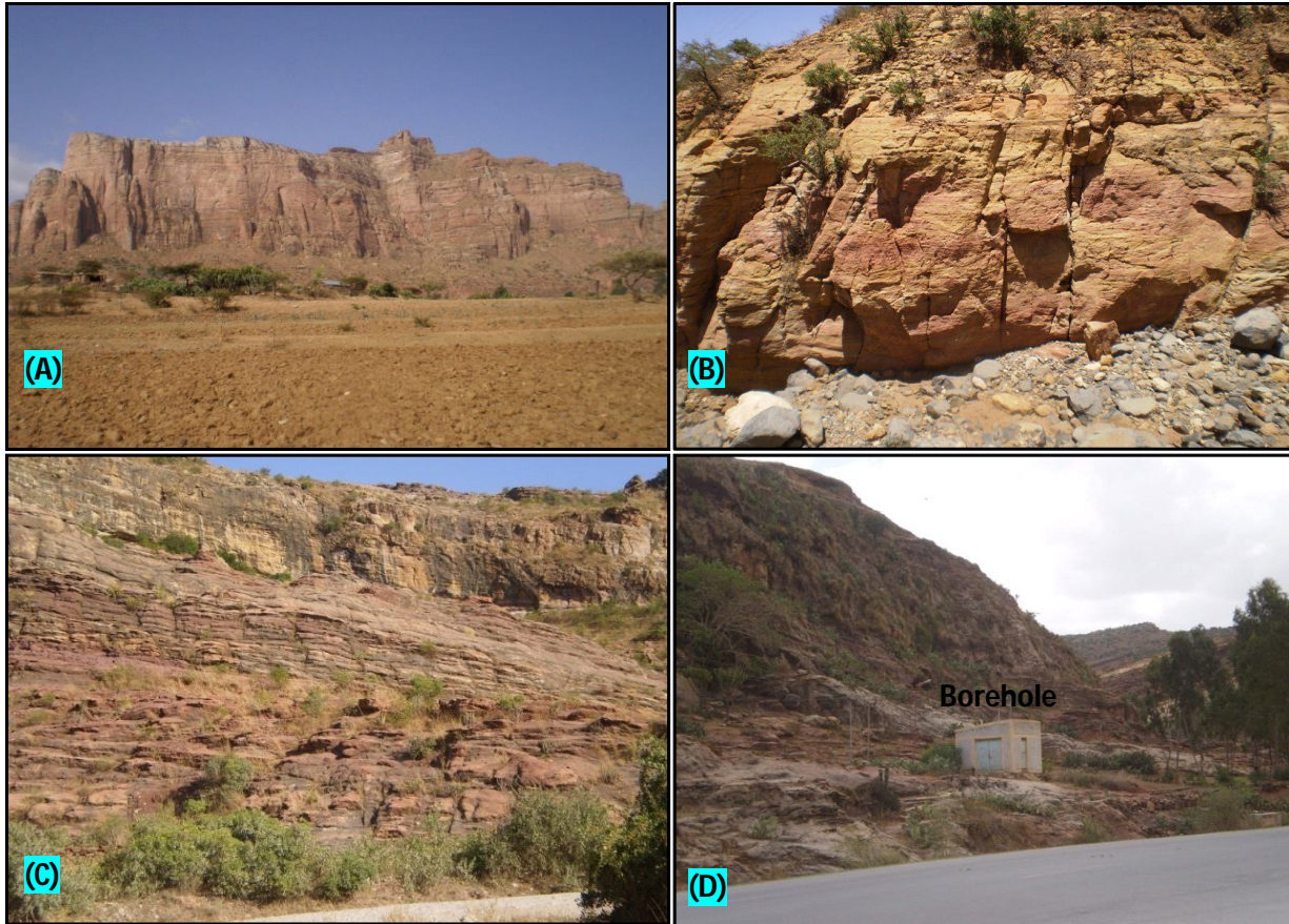
Fig 25 Hill of Adigrat Sandstone near Megab (Hawzien) (a), closer look into exposure of the Adigrat Sandstone (jointed gravely-sandstone) near Agibe (b), hill side exposure of jointed sandstone near AbrihaWeAtsbiha (c), water supply borehole drilled in to the Adigrat Sandstone in Wukro (d)
