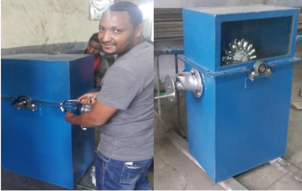
Figure 3.24a: Photography of fixing of upper casing Figure 3.24b: Final product
