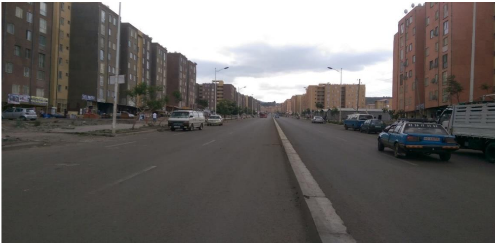
Figure 3.2. Yeka Abado Condominium Site, (taken by the researcher)
