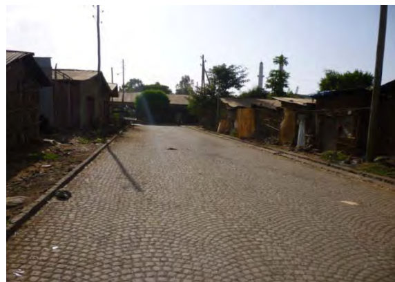
Cobble stone cover for internal roads
